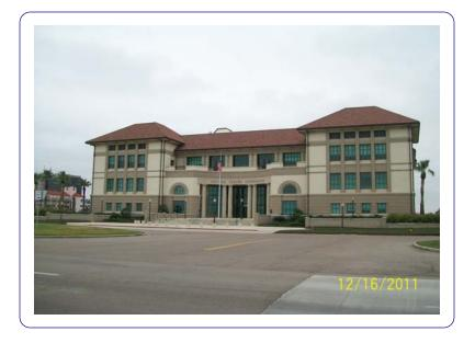
The U.S. Federal Building is located on Shoreline Drive in Corpus Christi, Texas. The building was constructed in 1997 and is generally comprised of structural steel framing. The roof consisted of two types of construction including a low-sloped modified bitumen roof and steep-sloped clay S-shaped tile roofs. Leaks were experienced in the tile roof areas almost since original construction.
