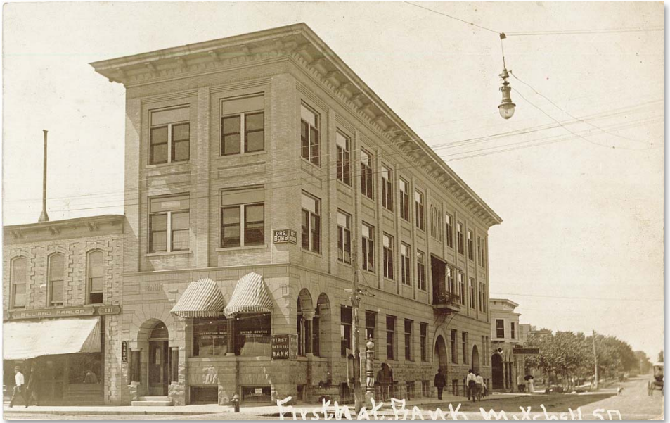
Originally built as: First National Bank (1906) FIRST NATIONAL BANK 123 North Main Street
