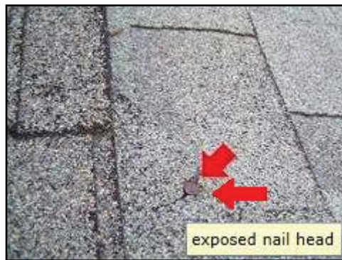
3. Exposed fasteners
