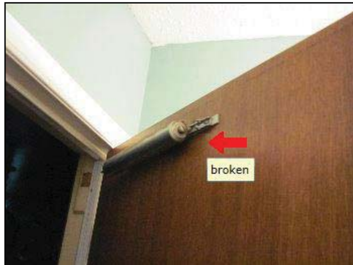
8. self-closer damaged
