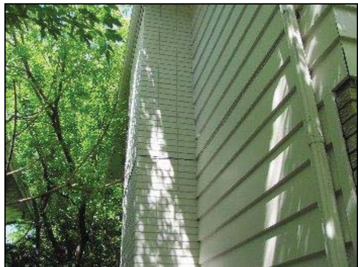
10. trees close to building
