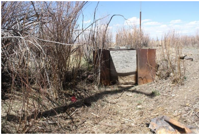
Headgate looking downstream
