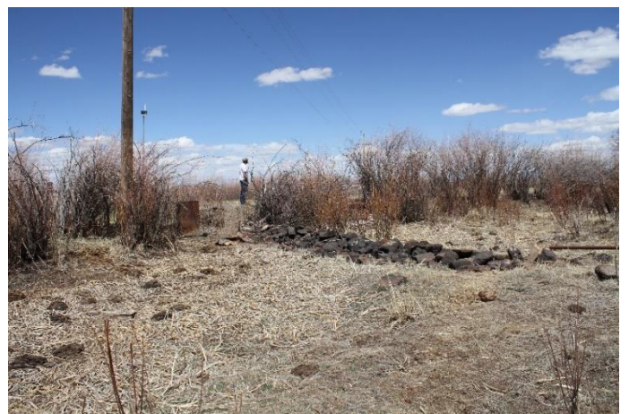
Headgate and diversion dam
