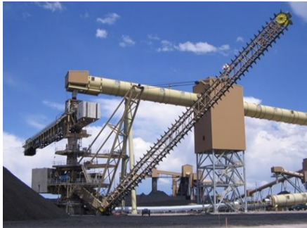
Bulk Storage Technology
