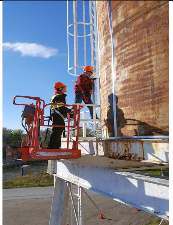
How to beautify this rusting structure? ...By covering it with stretched banner material
