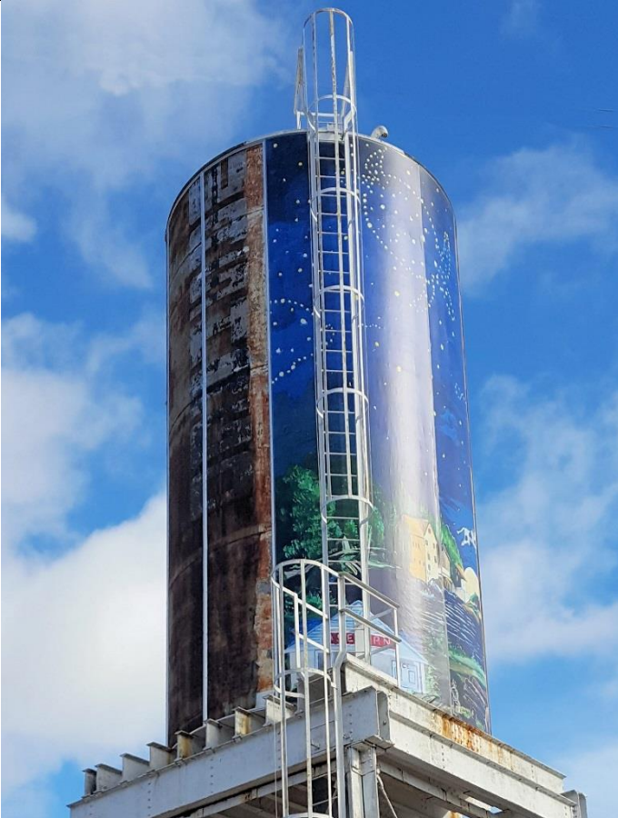
A very neat installation realized by Pixel N' Print, from Severn, ON Canada. www.pixelsnprint.ca
