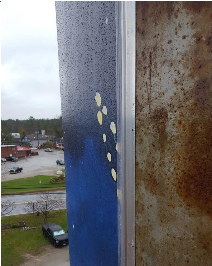
The first printed vinyl panel is installed
