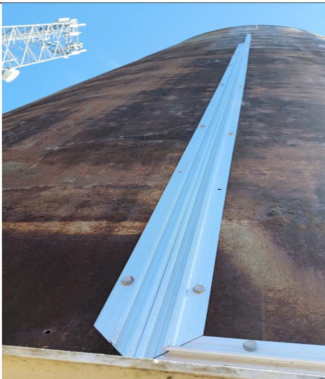
The TS23 was the chosen extrusion for this project
