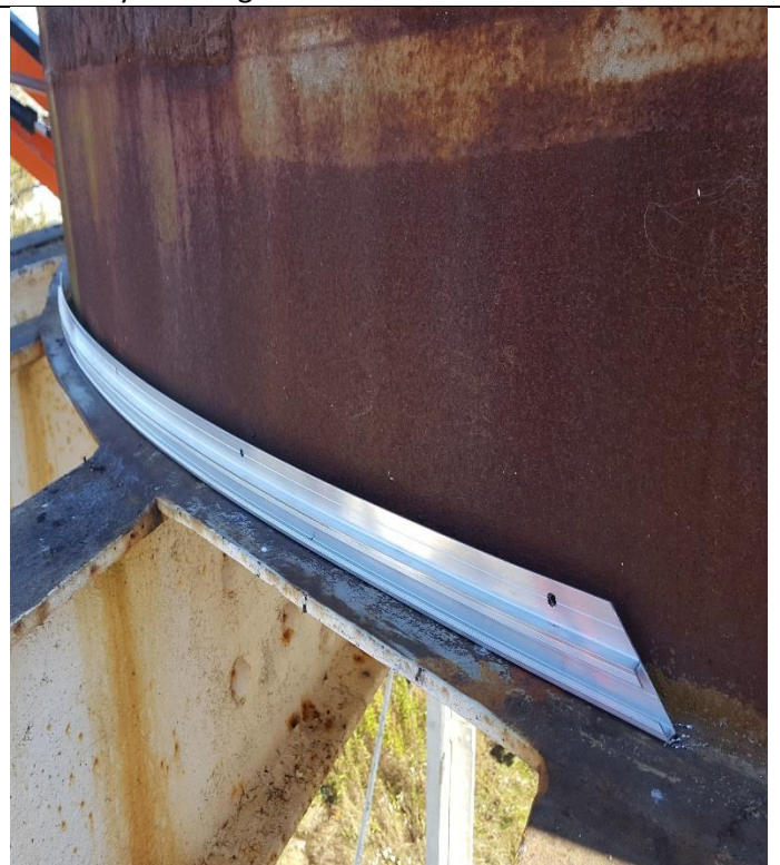
It can be bent to fit the curvature of the water tower
