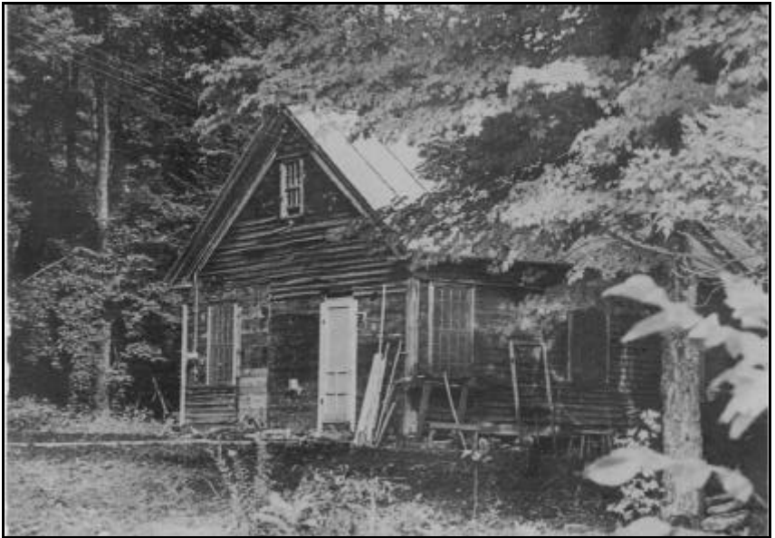
Schoolhouse #6 during remodeling efforts
