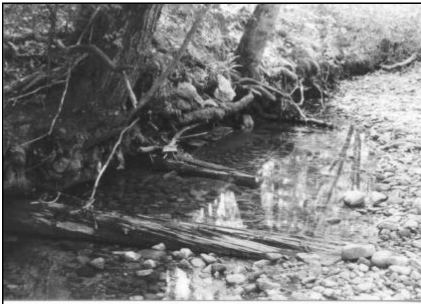
Hemlock logs laid across the brook in 1802 to support Batchellor's dam
