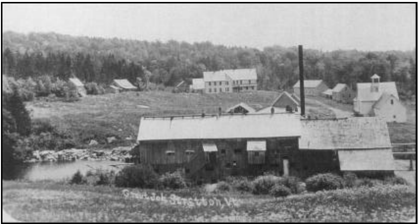
The Grout Job as seen looking east along the Stratton-Arlington Rd. The mill sits directly over the river.
