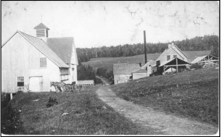
The Grout Job as seen looking west along the Stratton-Arlington Rd.
