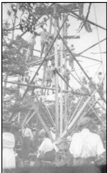
The Tower under Construction
