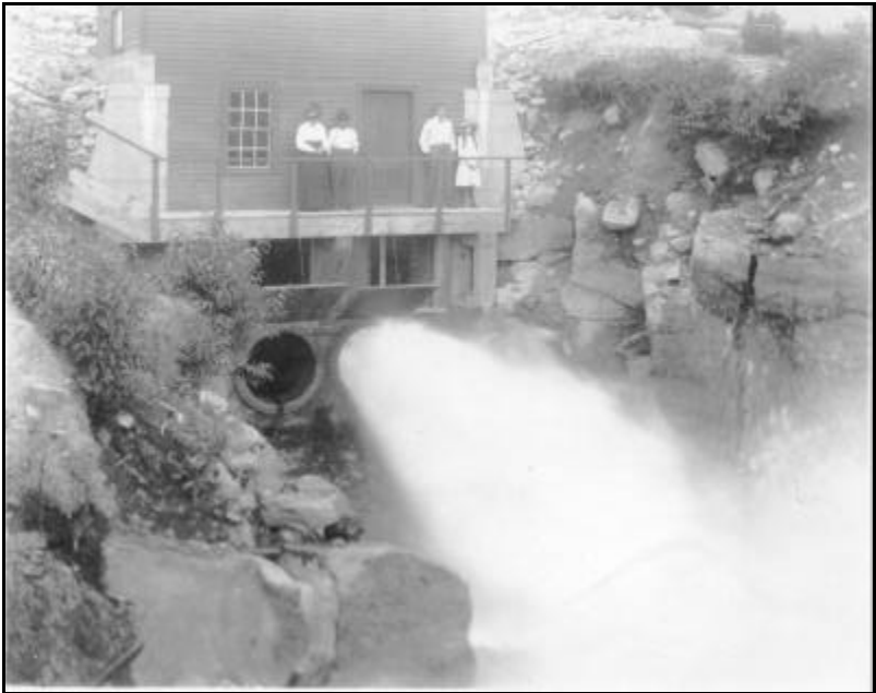
The Discharge Station Inez, Elmer, Hermon and Doris Eddy on the platform
