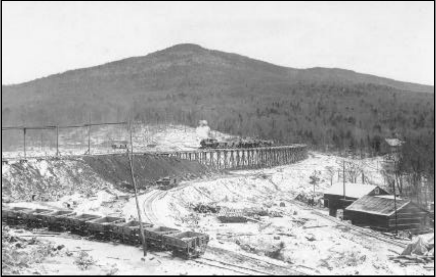
Dam construction with Mt. Pisgah (Mt. Snow) in the background
