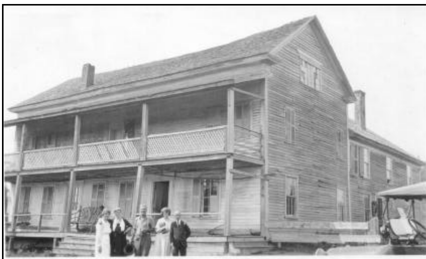
The Kelley Stand Hotel in Sunderland in the 1920s The man in the center is Robert Lawler, a squatter who lived in the old abandoned hotel.
