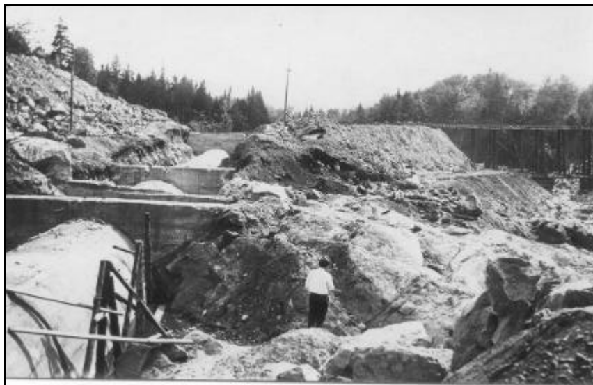
Piping from the Reservoir to the generators
