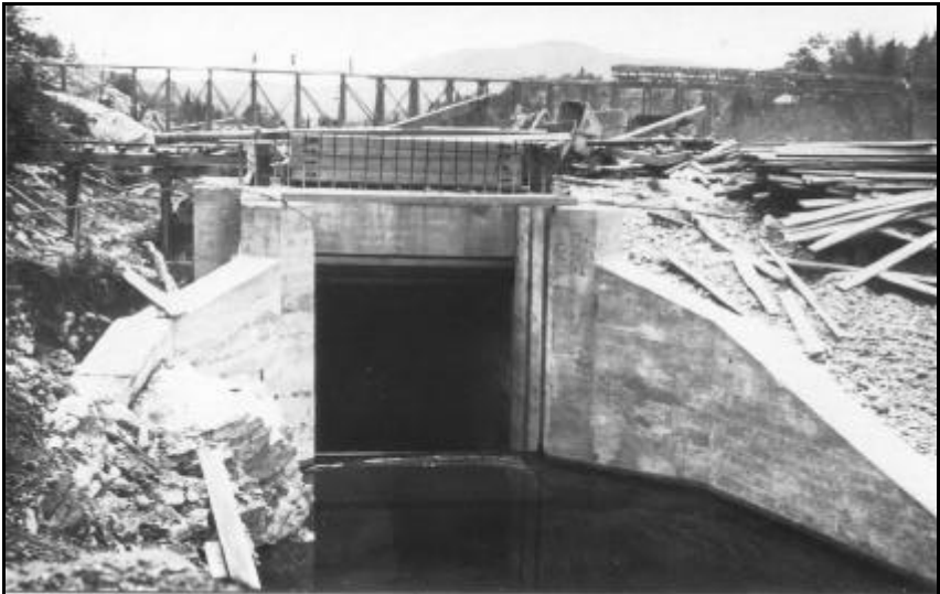
The intake side of the Discharge station (under construction)
