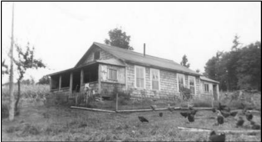
Lawrence Denker's house on the site of what is now 440 Stratton-Arlington Rd.
