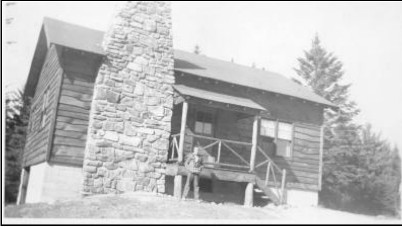
The Caretaker's cabin at Grout Pond This building was intentionally destroyed in 1999.
