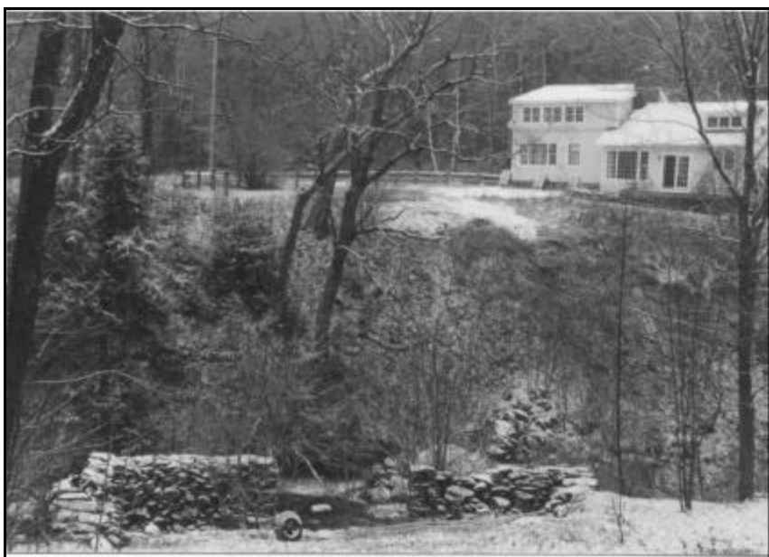
Remains of the Lyman Mill in Pike Hollow with 218 Penny Ave. overlooking the site
