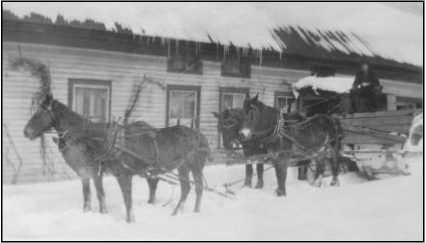
Winter roads were prepared by horse-drawn snow-rollers Although unidentified, this rig apparently was Stratton's snow-roller.
