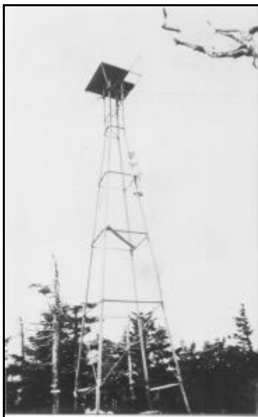
The Tower A later photo from 1930
