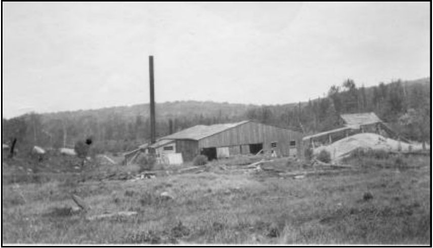
The Mill at the Dufresne Job
