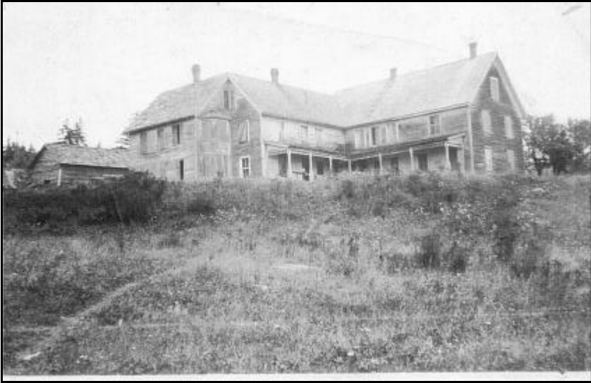
The Boardinghouse at the Grout Job
