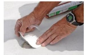
Note: Make sure all surfaces are clean, dry and free of oil or dirt when applying tape. Use a nonresidual solvent to remove oil or grease on the surface to be taped. Residue can create a chemical reaction effecting the tape adhesive. Take care to allow the surface to dry fully before application of the product.
