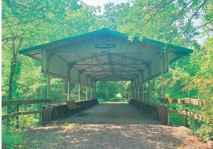
Photo 7 Bridge over County Road 20-40 (Liberty Street)
