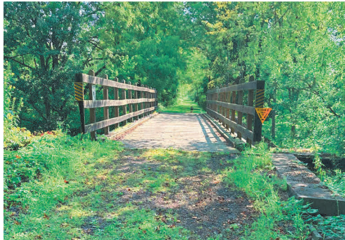
Photo 6 Bridge over Beaver Creek
