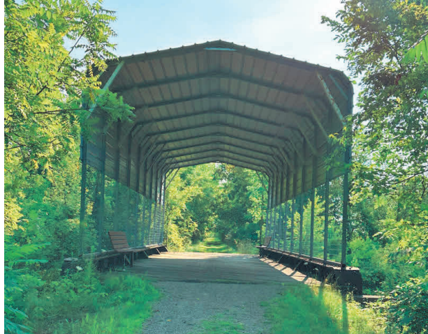
Photo 5 Bridge over County Road 15
