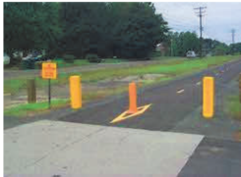
Photo 10 Bollards at Access Points
