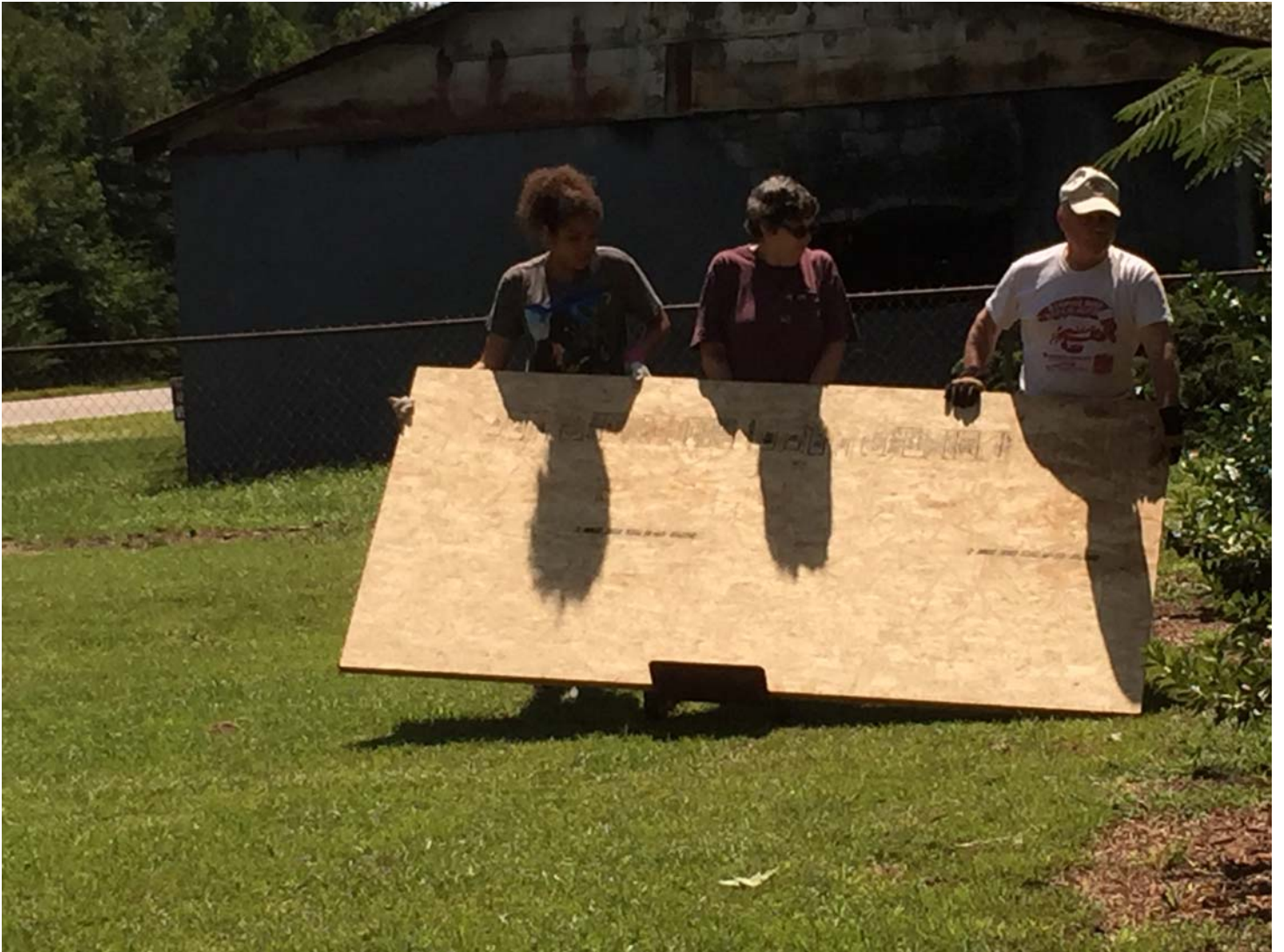
Moving plywood that will become part of the new subfloor.
