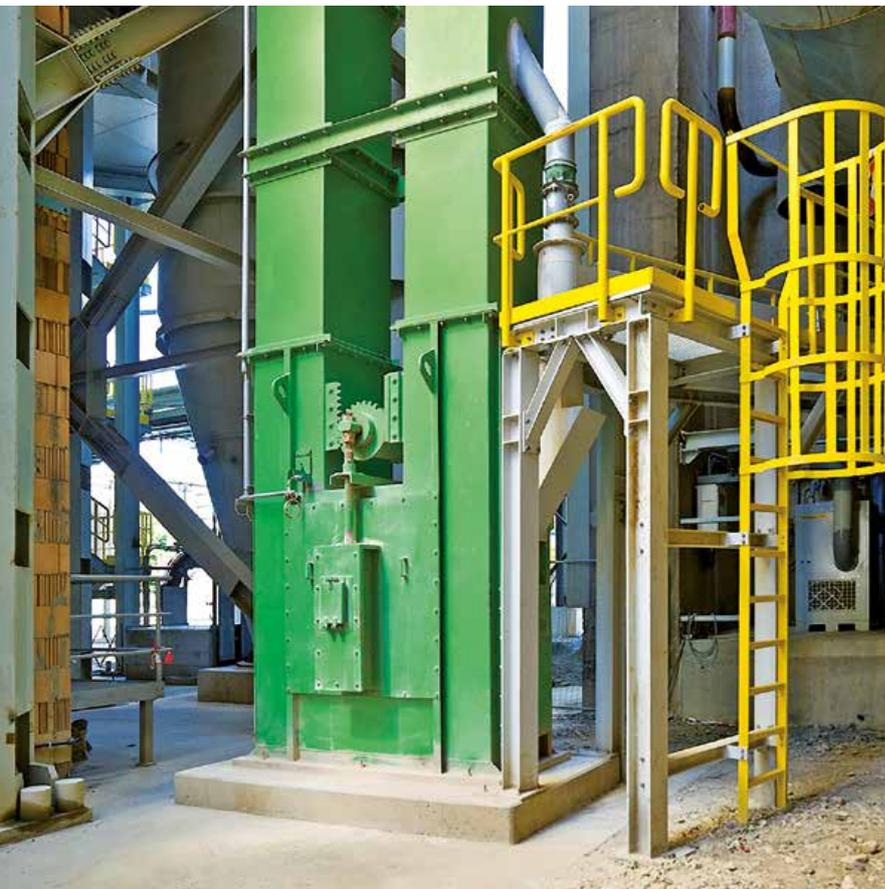
Elevator boot with parallel tensioning device
