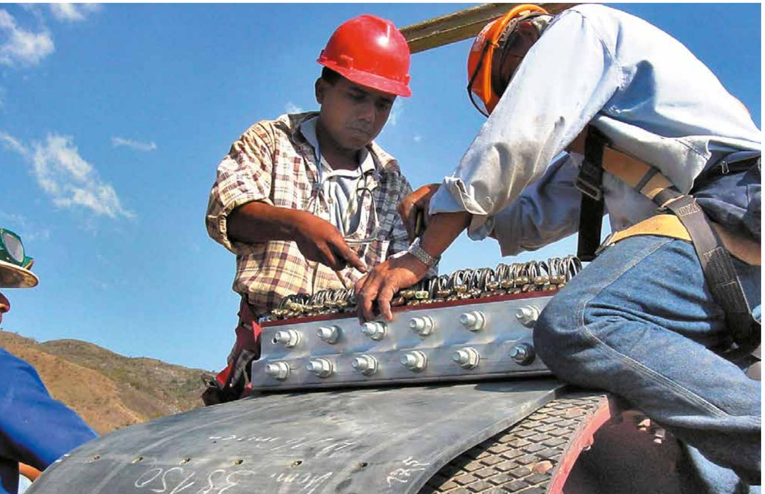
Splicing of steel-reinforced belt
