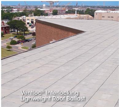
Ventloc® Interlocking Lightweight Roof Ballast
