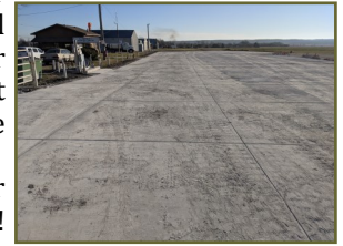
Airport Taxiway - After
