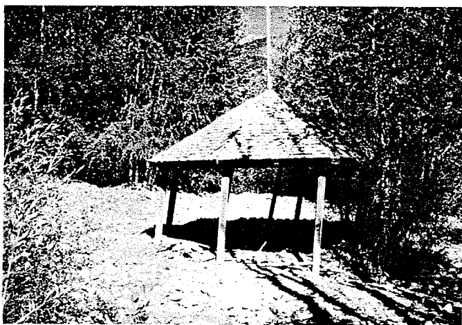
Fig. 8 — Top of two level park bandstand in town of Marble. Lower part was buried by mudflow debris of 1945 Carbonate Creek flood.
