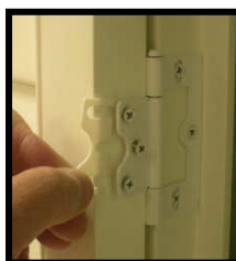
Insert hinge spacer.
