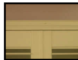
Double check panels before securing.
