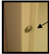
Only secure one screw into the bottom left frame.
