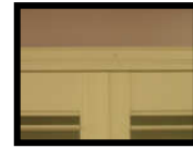
Double check panels before securing.
