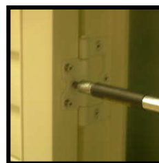
Tighten screws.
