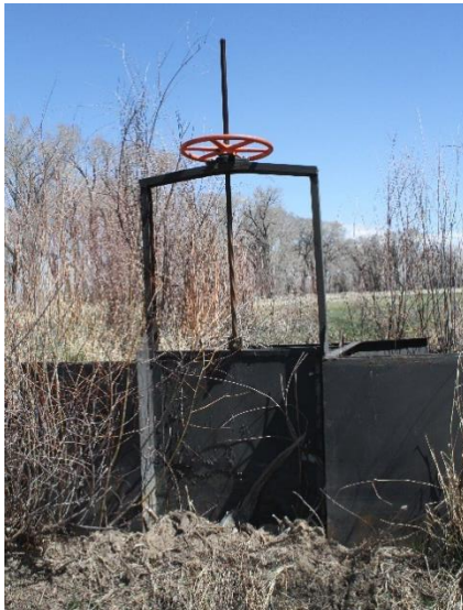
Headgate looking downstream
