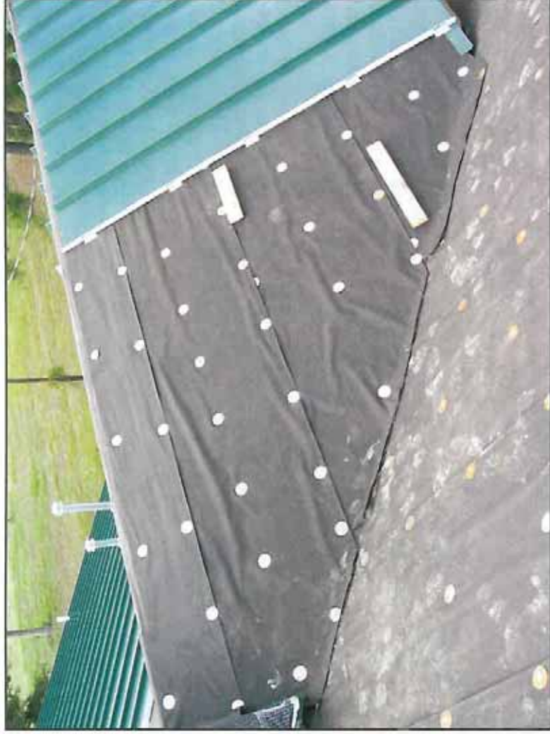
Typical wrinkled organic felt underlayment.
