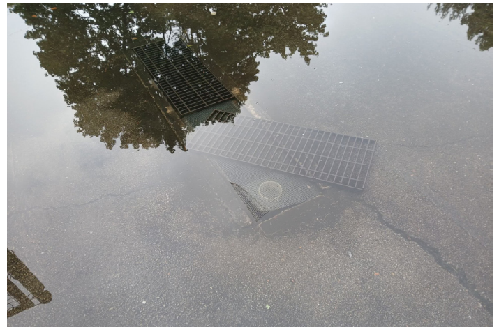
8 inches under water 16 hours after the rain
