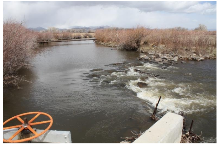
Headgate and diversion dam
