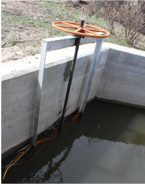
Headgate looking downstream
