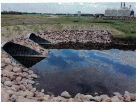
3-Culvert Hwy 45 & 29.jpeg 485K
