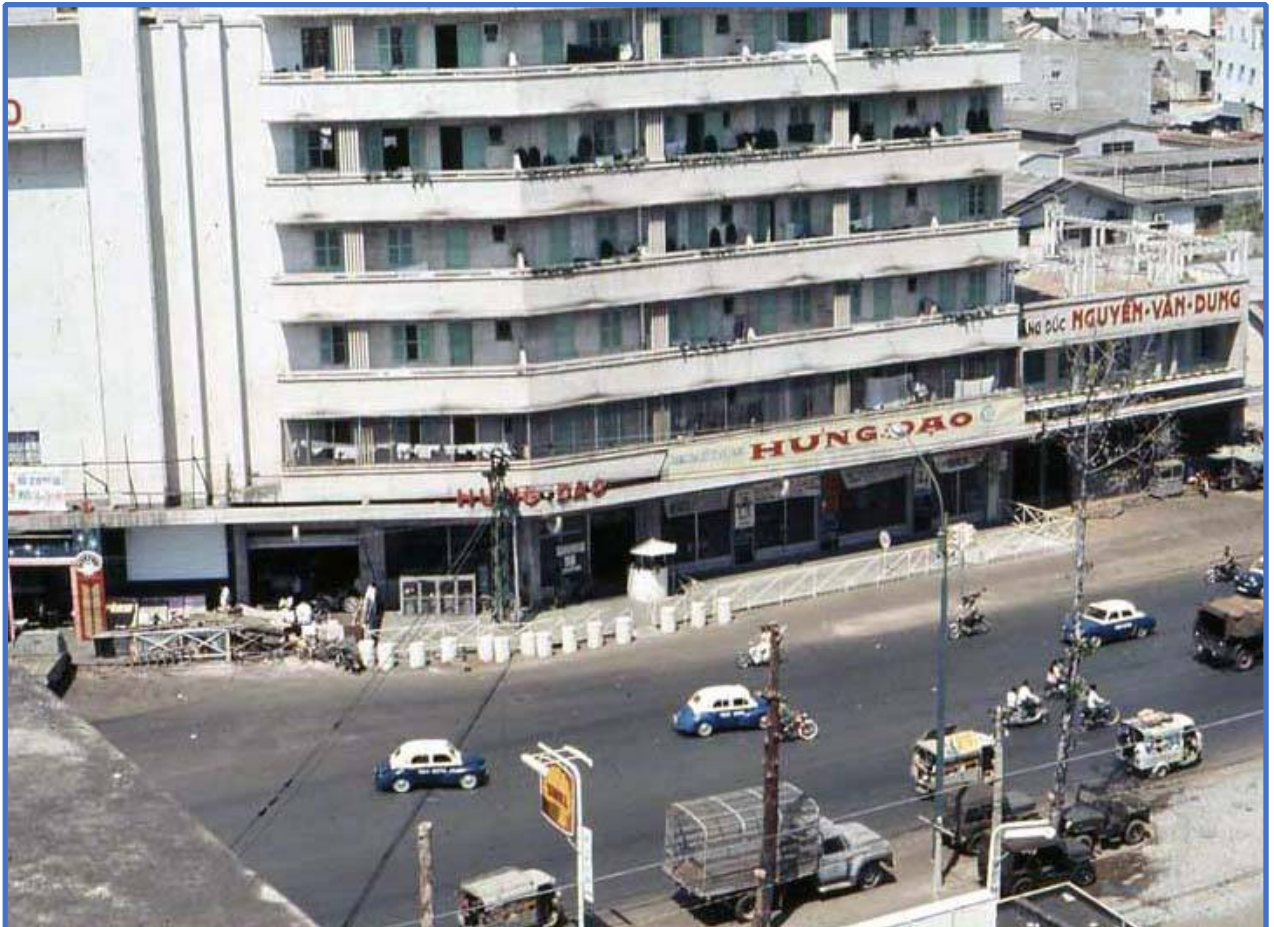
The Hung Dao BEQ as seen from the Ky Son Annex BEQ roof.
