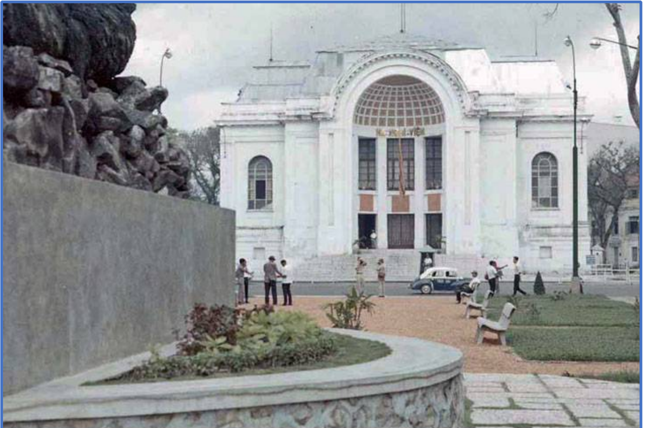
The National Assembly Building. The lighter part of the roof on the right shows where it was repaired after a rocket hit the building in September 1968.
