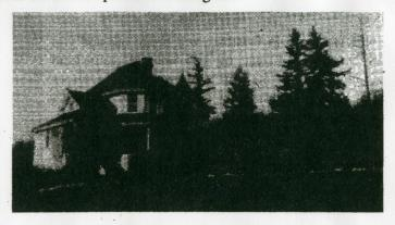
The resulting structure was a two-story Queen Anne Style building featuring shiplap siding and a wood-shingled hip roof with a turret dormer. A porch with a whimsically decorated railing was added along the south elevation. The first floor consisted of three main rooms (dining, living, study), an entry hall, bathroom, modified kitchen and pantry. Four bedrooms were constructed upstairs. A central chimney heated the house through an elaborate system of stovepipes.
