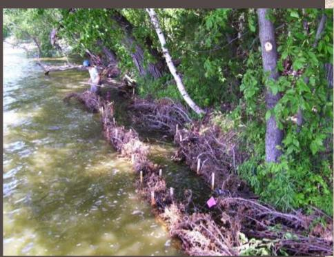
Brush Bundles being installed with 4 foot hardwood stakes
