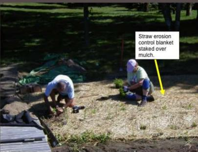
If high water or flooding is possible, a straw erosion control blanket is staked over the mulch prior to planting to prevent the mulch from being washed out. The blanket should have bio-degradable netting. Synthetic photo degradable netting often lasts many years and animals can get caught in the netting.
