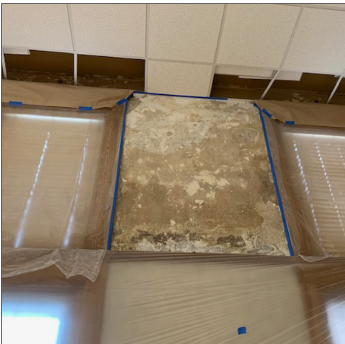
The work has started on the south wall in the gallery.
