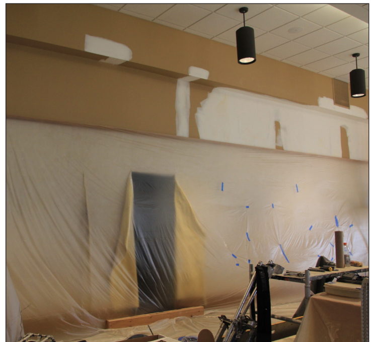
Gallery east wall – Ready for painting. (More pics page 10-11)
