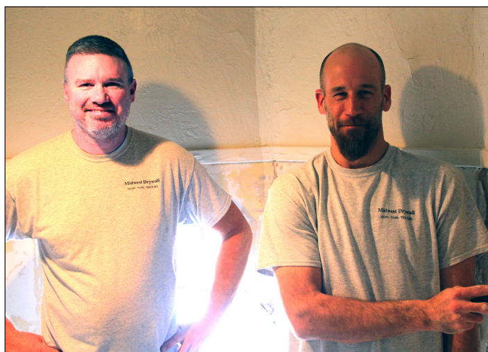
Travis Kelly and Andrew Thu from Midwest Drywall working in the bathroom.
