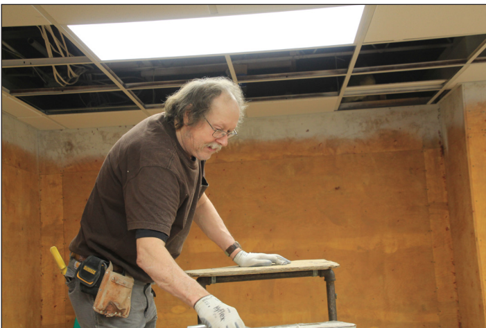
Gary Sandness replaced the old ceiling tiles made of plywood with white ceiling tiles. This should make the room lighter also.
