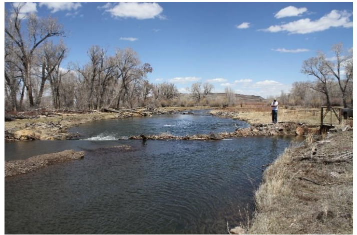
Headgate and diversion dam
