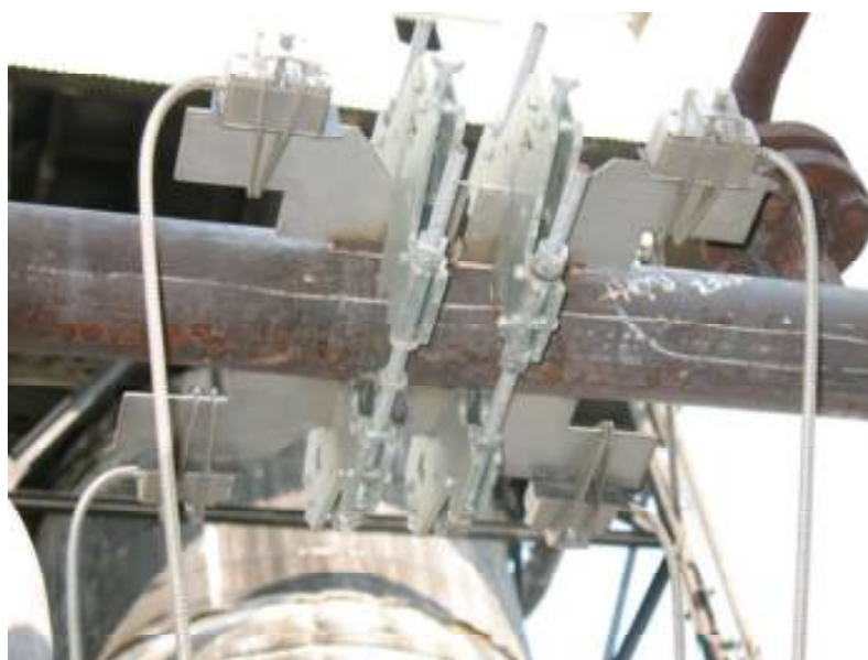
Fig. 18 : Final Installation Prior to Lagging
