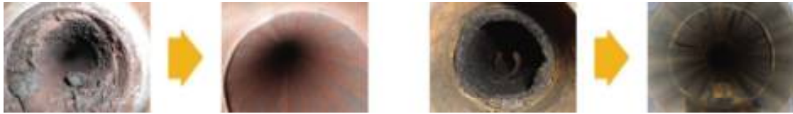
Fig. 25 : Before and After Decoking by Pigging [7]
