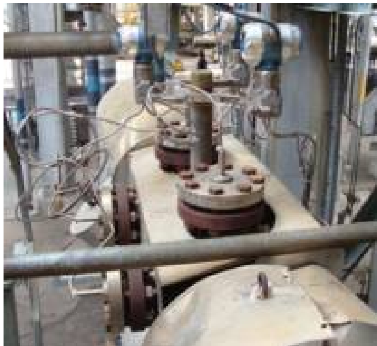
Fig. 3 : Wedge Flow Meter on Coker Feed Using Three DP Transmitters with Diaphragms
