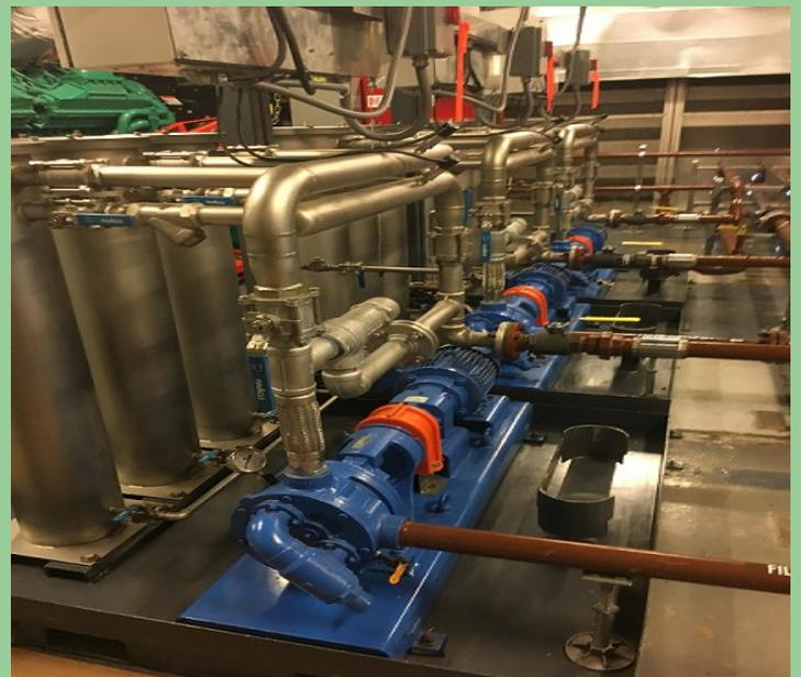
( Above is the RSI 100 Gpm, this unit is location in one of the largest USA telecommunication company's data Center in North America. It is insuring the best fuel quality for 1 million plus gallons . These systems shown above polishes the fuel before in enters the tanks, fuel can also be transferred from tank to tank with polishing as needed )
