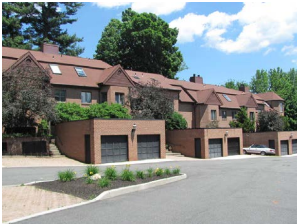
Building front elevation and detached garages
