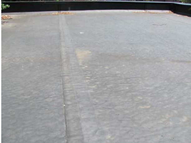
EPDM roof at garage
