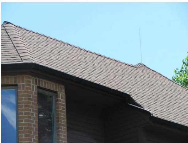
Laminate shingles at Building 3
