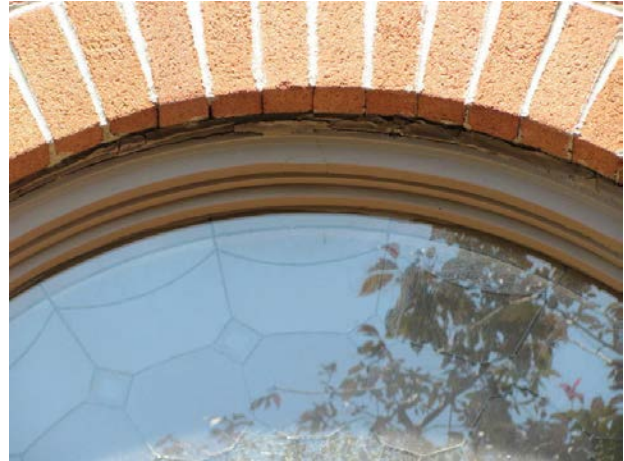
Sealant cracks
