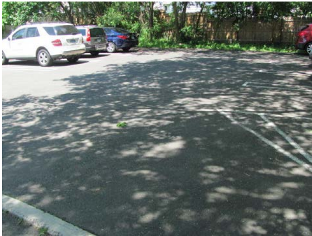
Asphalt pavement parking area
