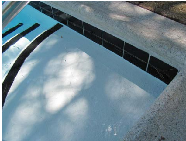
Pool finish in good condition
