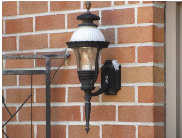
Finish deterioration
