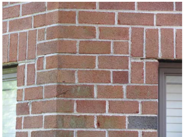
Mortar cracks
