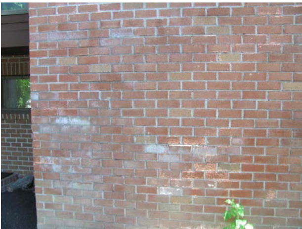
Efflorescence
