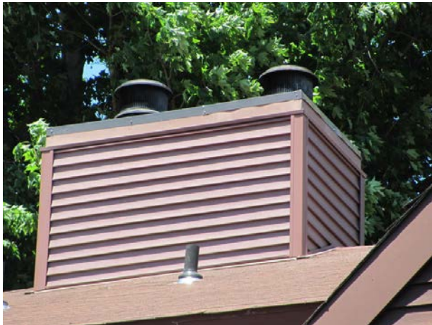
Typical newer chimney cap
