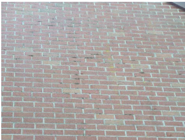
Mortar deterioration
