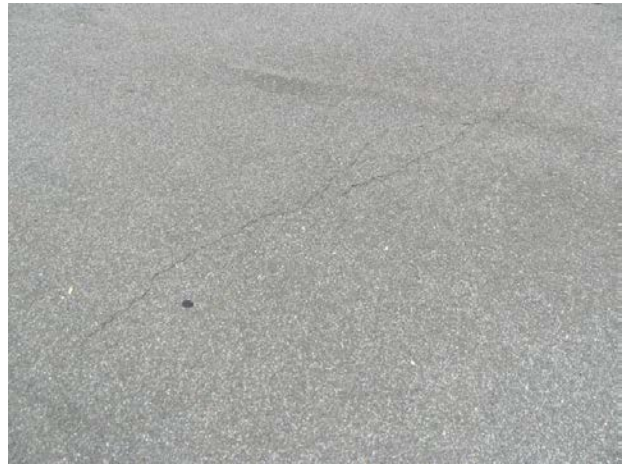
Minor crack
