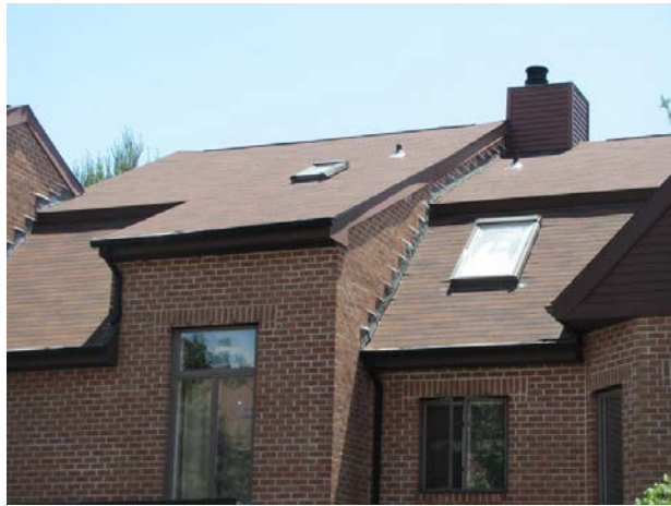
Replaced roofs at Building 1
