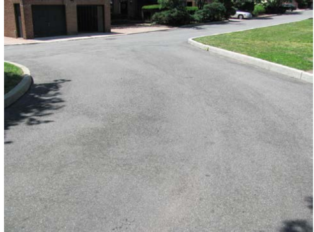
Asphalt pavement street
