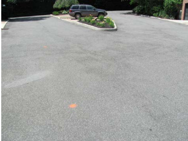
Asphalt pavement street
