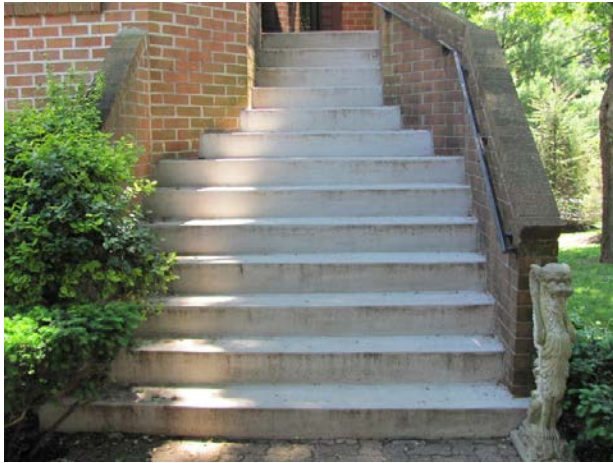
Newer concrete stairs
