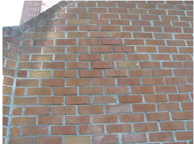
Mortar deterioration
