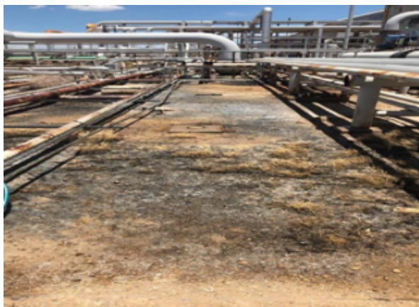
FIG. 6 – TWENTY-FOUR (24) HOURS POST TREATMENT WITH R3MEDIATE. WEST TEXAS GAS PROCESSING PLANT. HYDROCARBON RELEASE WITH SOIL, PIPE & GRAVEL STAINING. (R3ICS, LLC 2019 JULY)
