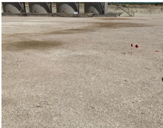
FIG. 3 – HYDROCARBON RELEASE ON OPEN AREA OF CALICHE PAD SITE IN WYOMING (R3ICS, LLC. 2019 JULY)
