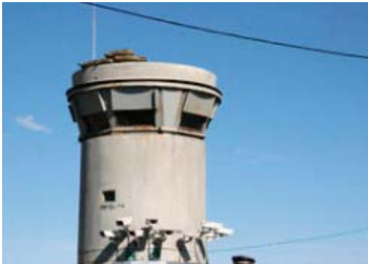
B. Motorola cameras on watch towers in the West Bank
