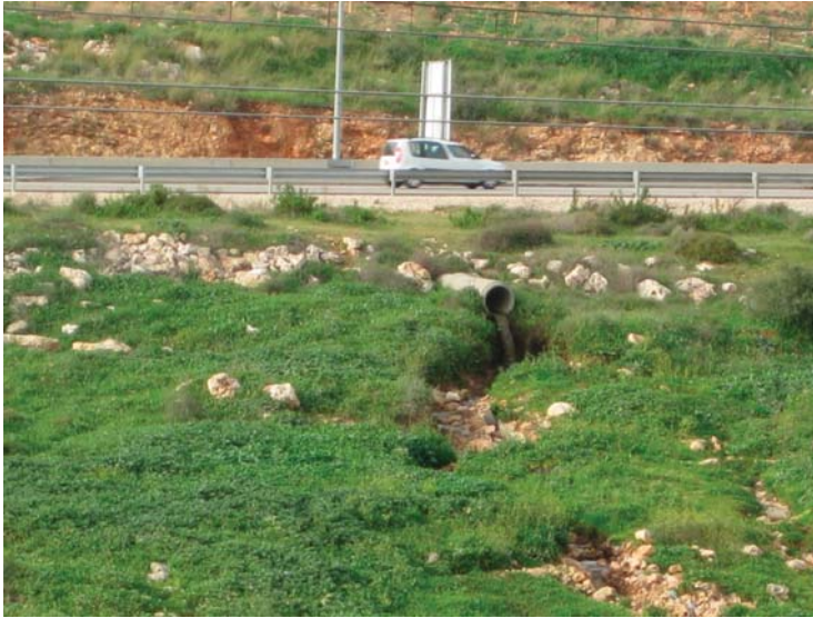
Brown untreated wastewater pours from an industrial zone near Barkan onto Palestinian land
