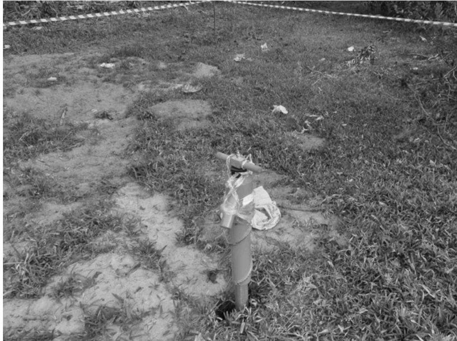
Figure 18. Borehole casing with Canzee pump ready for preliminary testing. Photo by author
