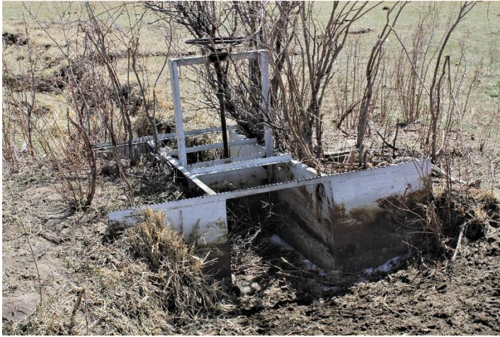
Headgate looking downstream
