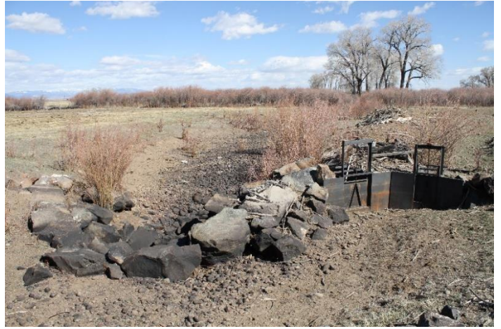
Headgate and diversion dam
