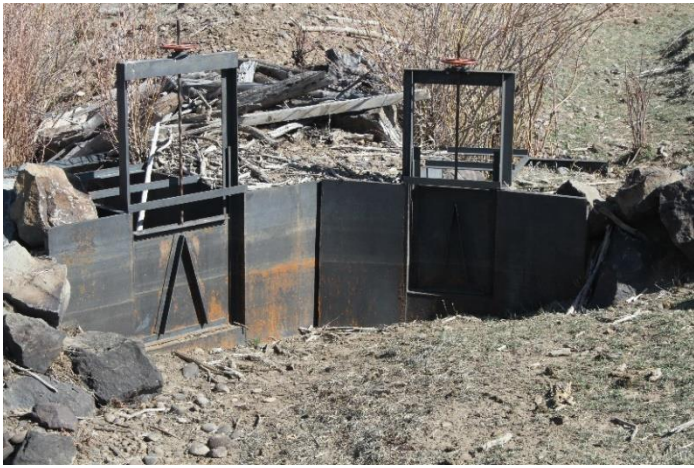
Headgate looking downstream
