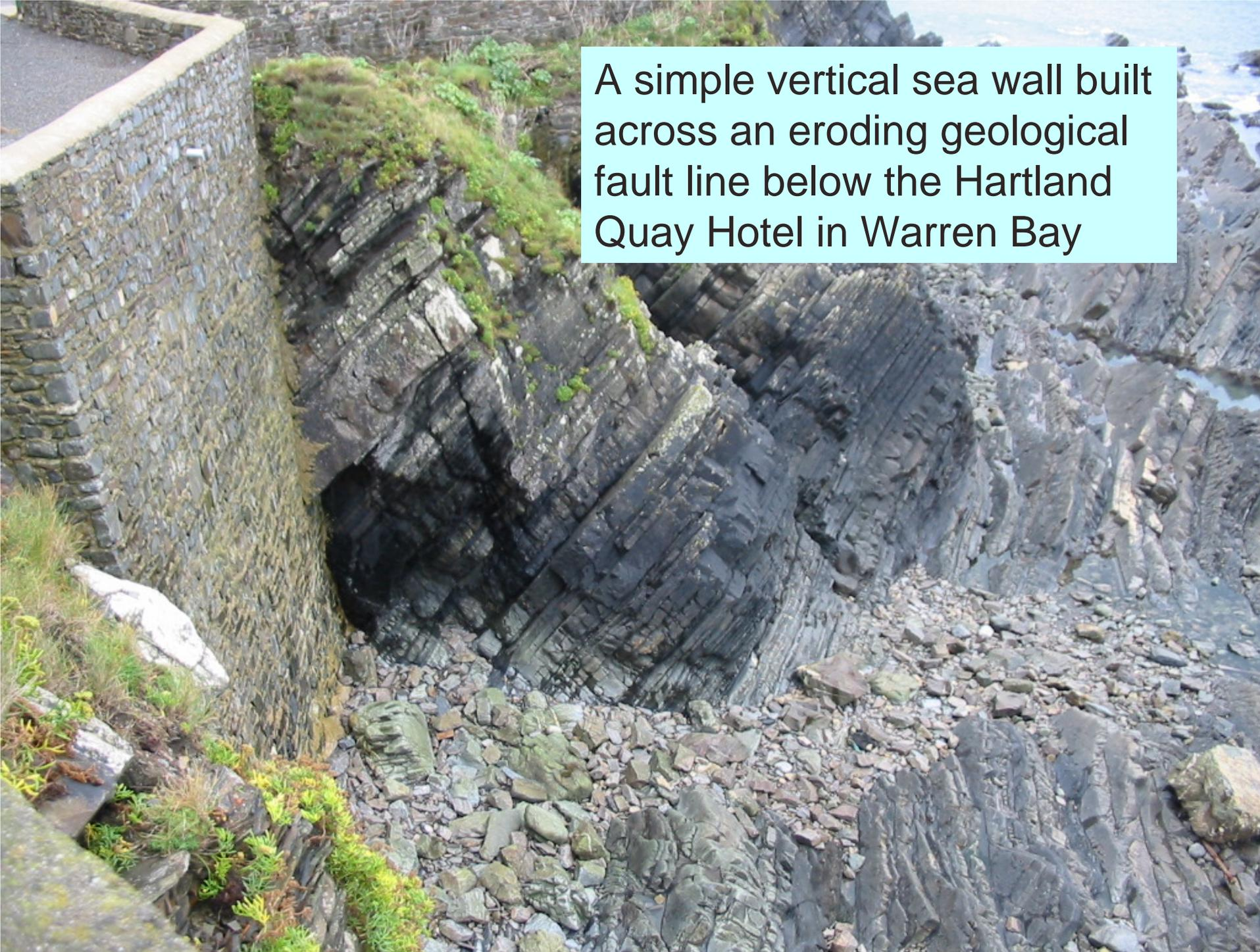
A simple vertical sea wall built across an eroding geological fault line below the Hartland Quay Hotel in Warren Bay
