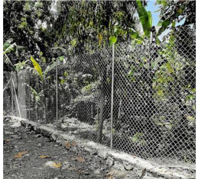
School of Barette, recess courtyard work in progress
