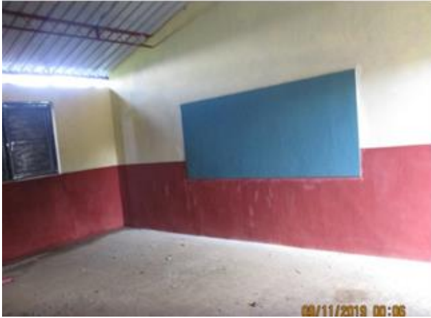
Inside a classroom, painting in progress
