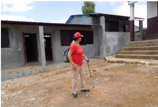
Construction site visit, May 2019
