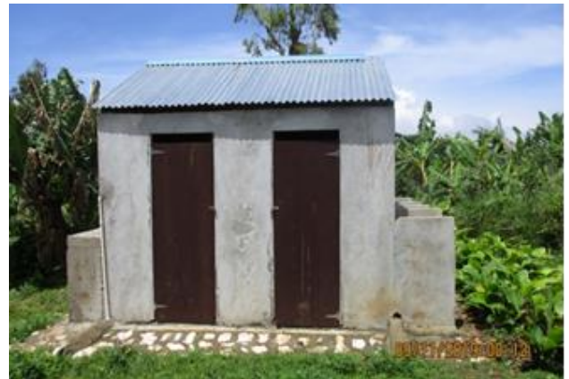
Restrooms, construction in progress
