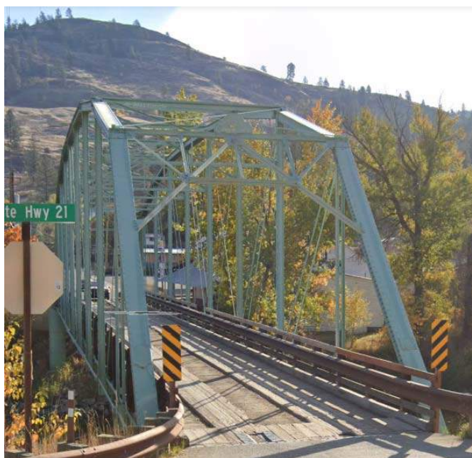
Wooden plank bridge in Curlew
