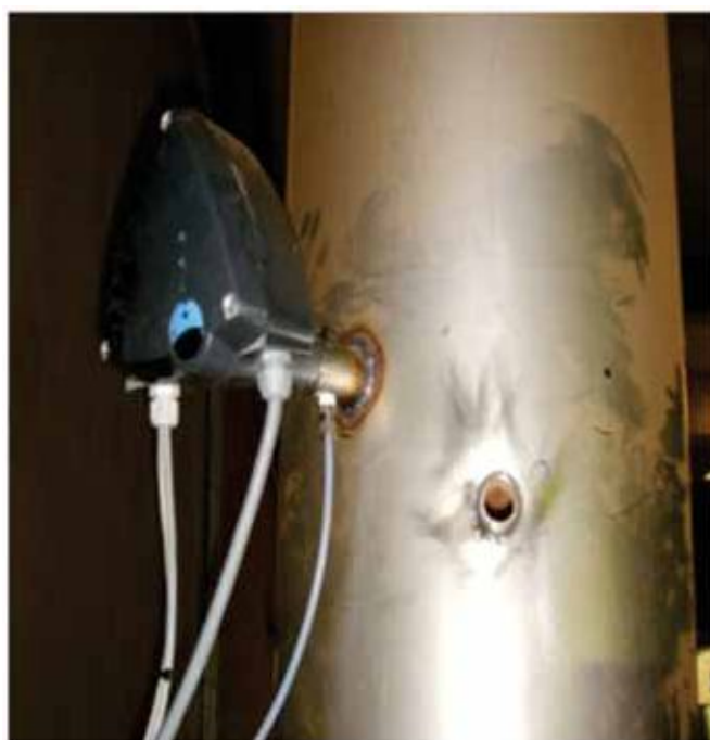
Picture 2. Installed triboelectric monitor (Sintrol Oy)
