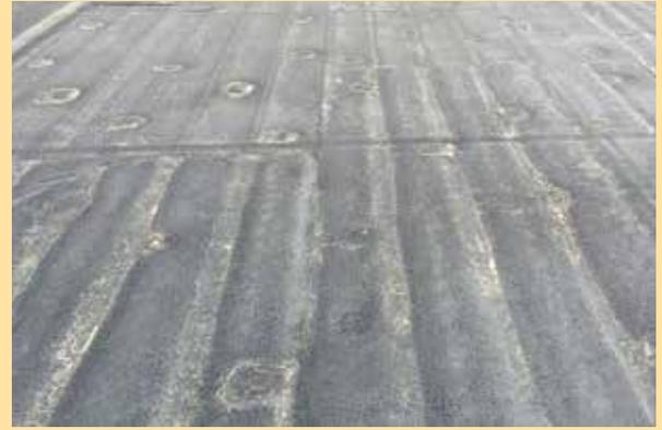
Example of rutting in polyisocyanurate insulation in an adhered EPDM membrane roof system
