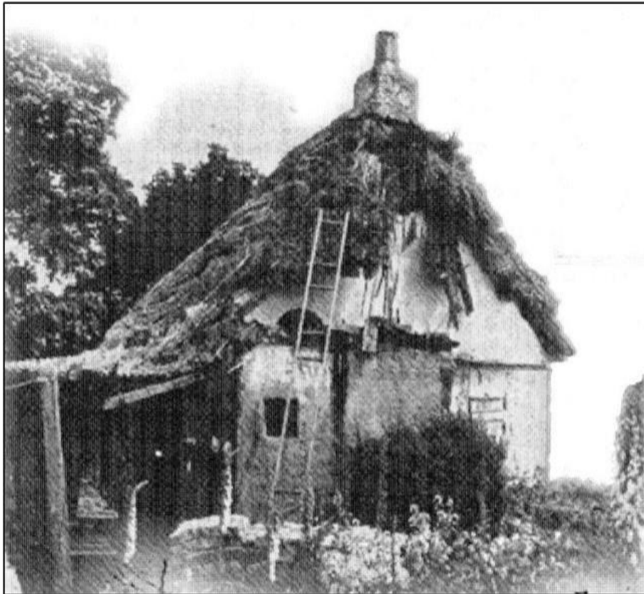
Some of the damage at the rear of the Roundhouse after the thunderstorm in June 1983
