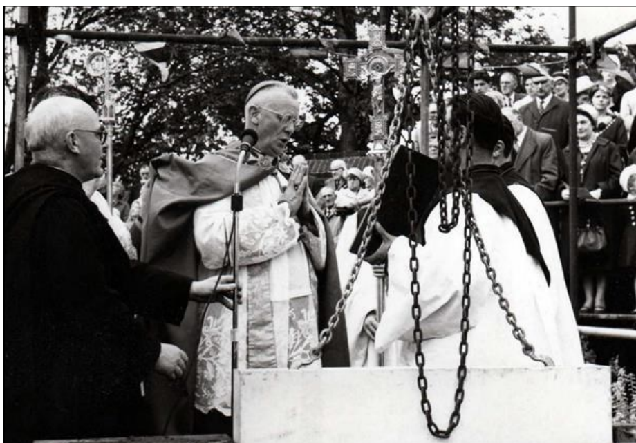
Father FitzSimons sees the laying of the foundation stone by Archbishop Heenan on 15 October 1962
