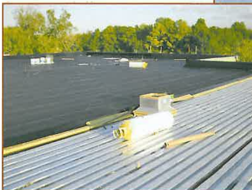
Photo 5 – Tie-in of modified bitumen on metal deck.
