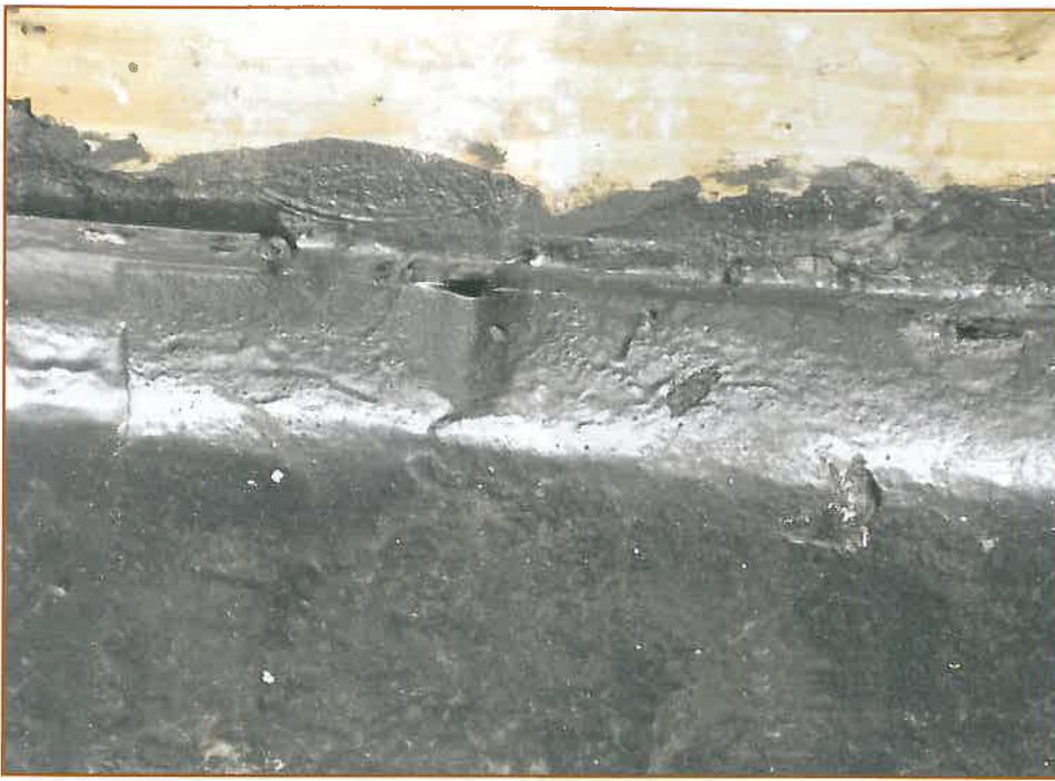
Photo 7 – Open fishmouth at top edge of felts.
