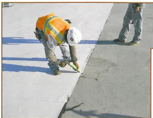
Photo 13 – Sealant applied along edge of fleece-backing single ply over lightweight insulating concrete.
