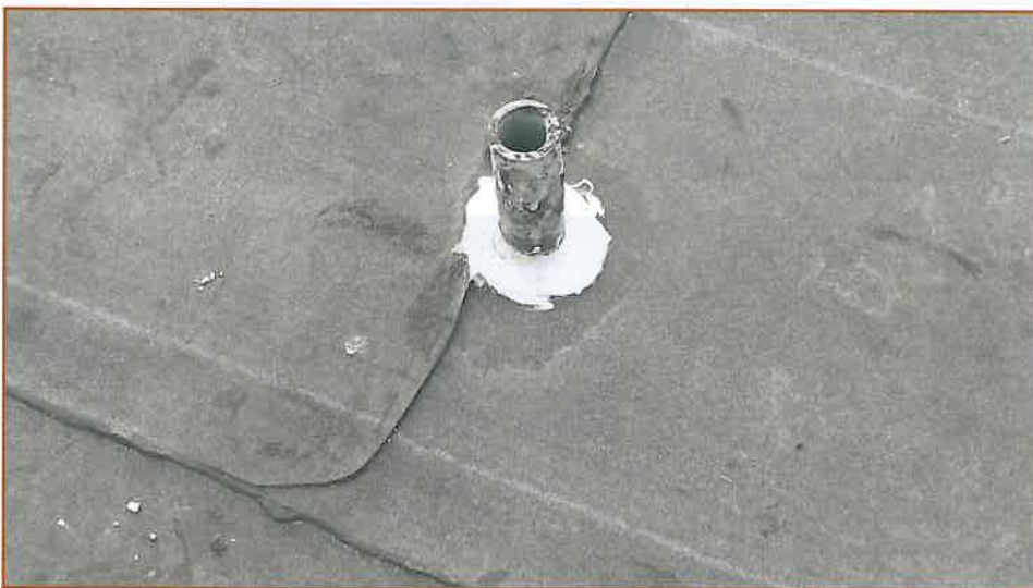
Photo 8 – Sealant applied around penetration on modified bitumen.
