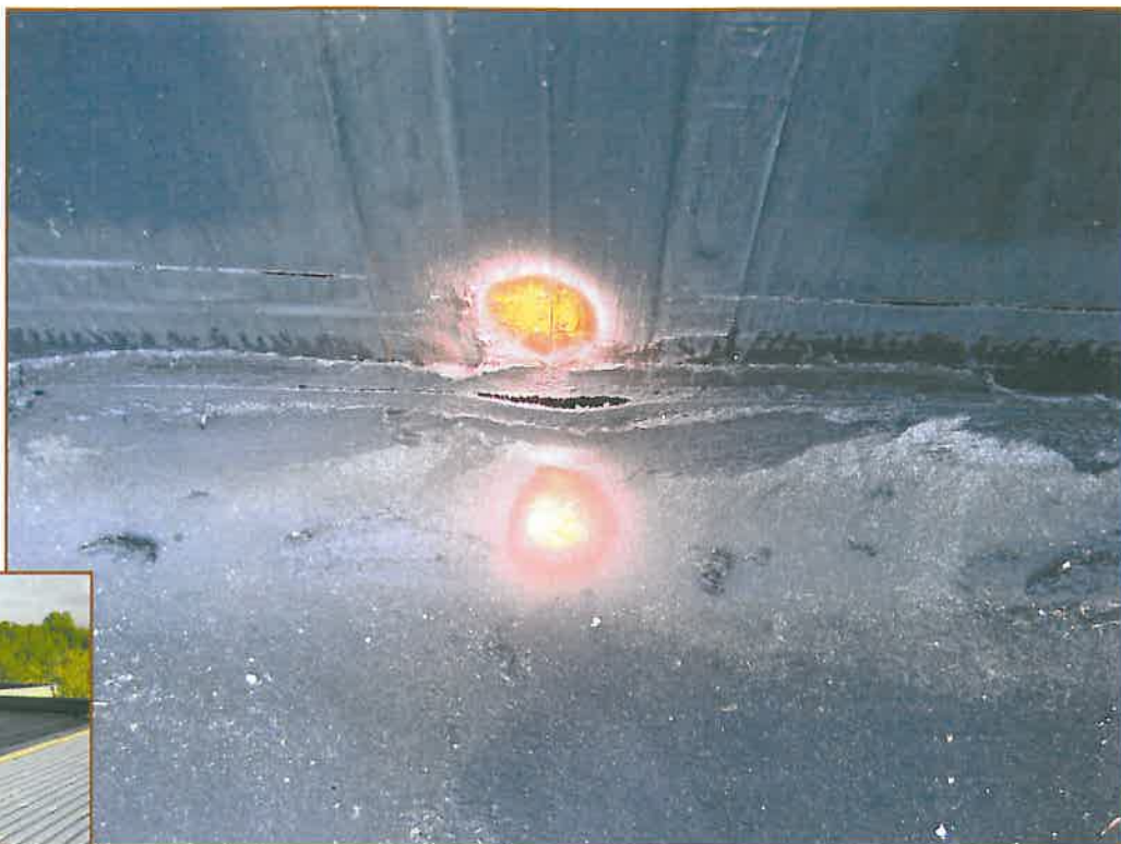
Photo 6 – Disbonded felts along parapet wall.
