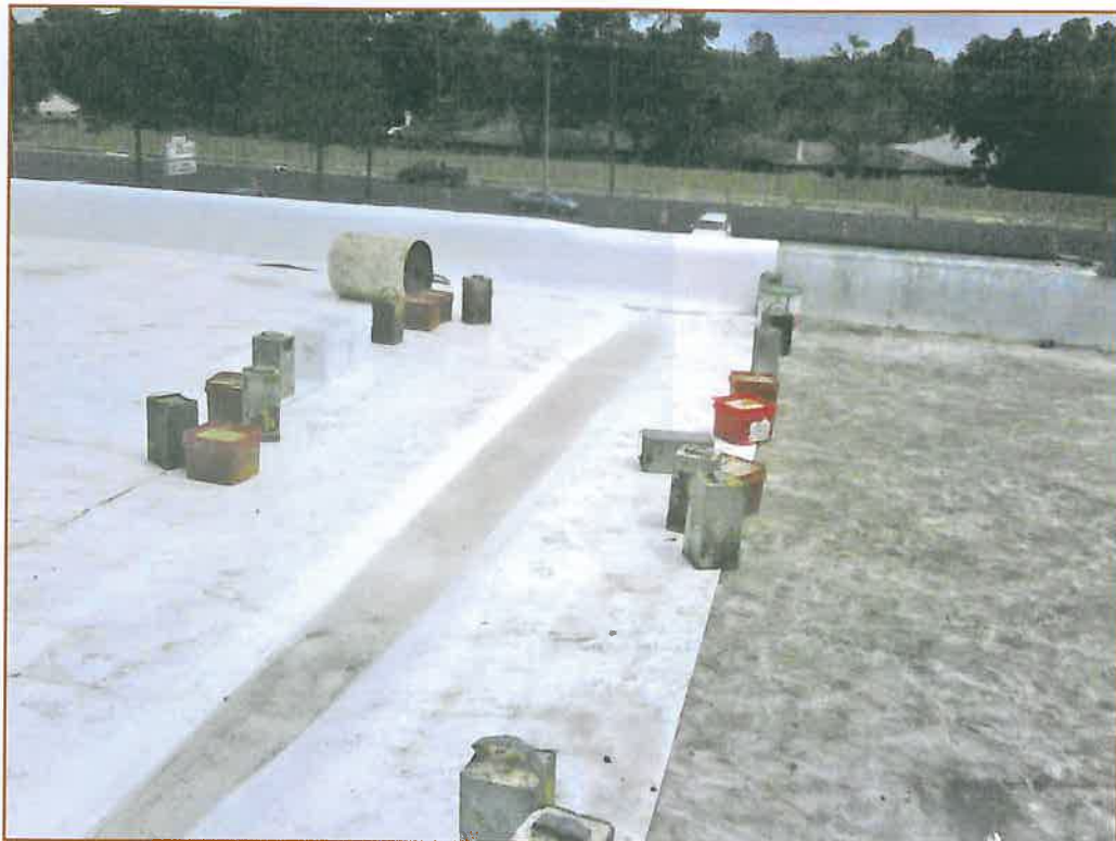
Photo 4 – Water accumulation on depression at tie-in.
