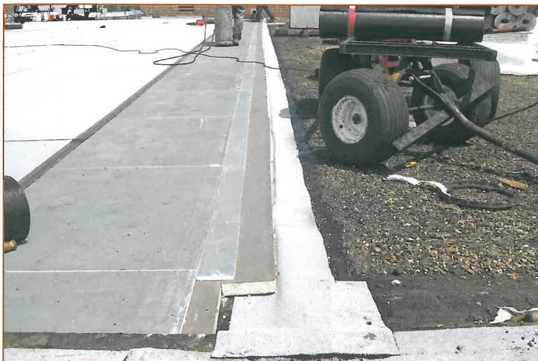
Photo 1 – Tie-in at deck and staggered insulation.
