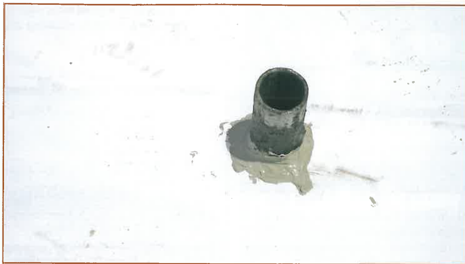
Photo 11 – Sealant applied around penetration in single ply as temporary seal.
