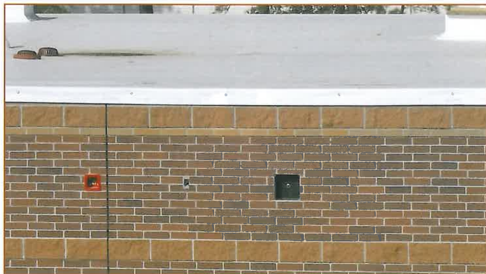
Photo 10 – Trimmed edge of single-ply at perimeter.
