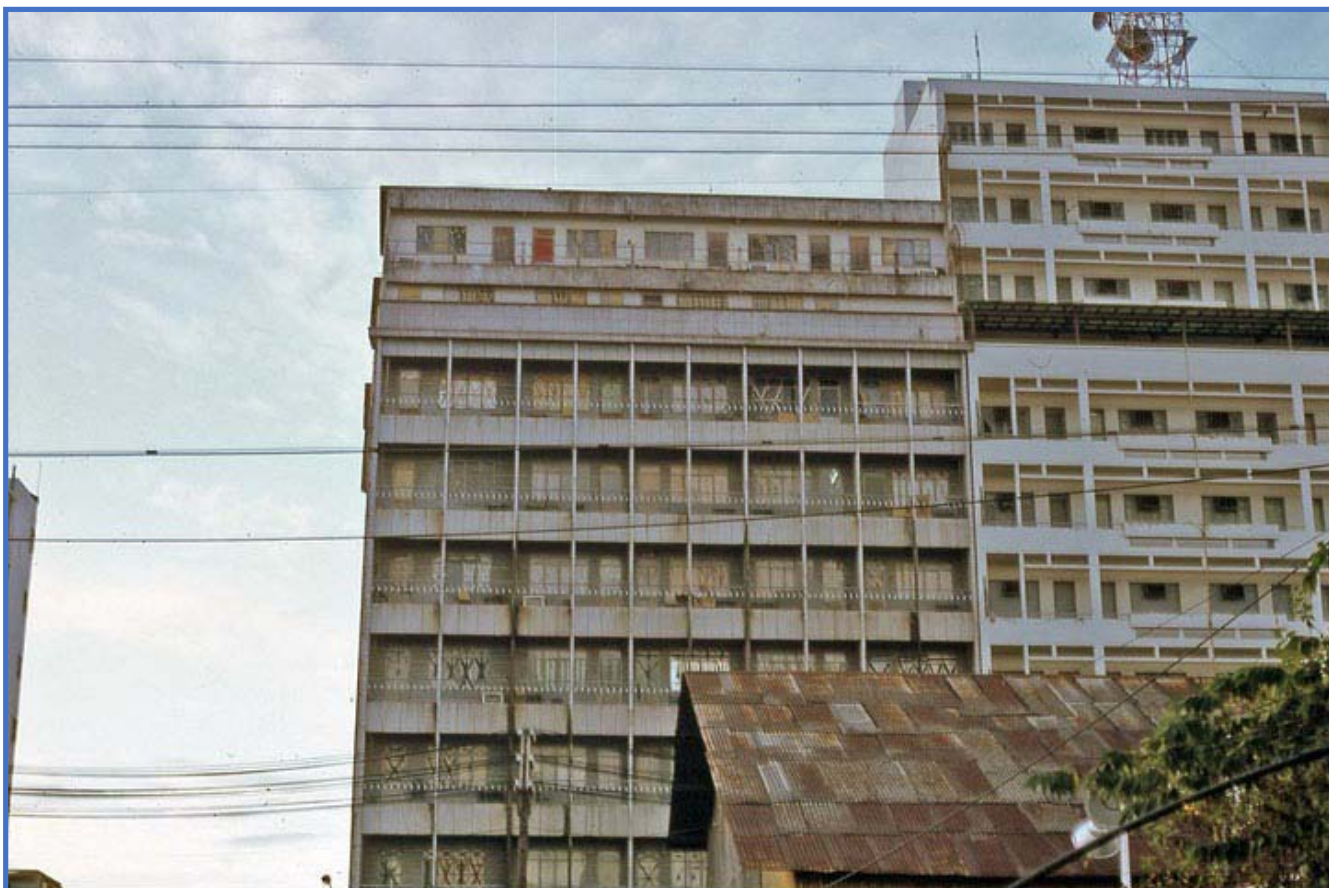
The Walling BEQ- the last BEQ used by the AFVN Saigon staff.
