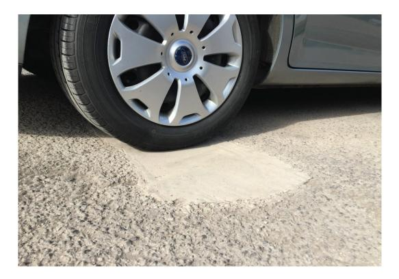
FastPatch 3-2-1 is a fast, effective way to quickly patch concrete and asphalt. Easily mixed and applied, simply add 3 parts powder to 1 part water (3-2-1). It is suitable for internal and external applications and ready for vehicle traffic in just 2 hours!
