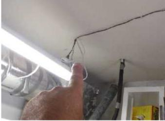
\* The use of extension cords for permanent wiring does not meet minimum building standards because the wiring within the extension cord is smaller than the house wiring which can increase the temperature of the extension wiring with potentially horrific event. The use of extension cords is for intermittent use only and not for permanent wiring. The use of extension cords for permanent wiring is a **SAFETY HAZARD CONDITION**.
