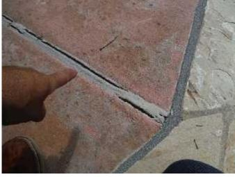
\* The separating and deteriorated elastomeric sealant between sections of the pool / spa surrounding concrete decking will allow moisture under the concrete decking which can cause the soil to expand eventually pushing the concrete decking upward. The separating and deteriorated elastomeric sealant is a patent **END OF SERVICE LIFE CONDITION**.
