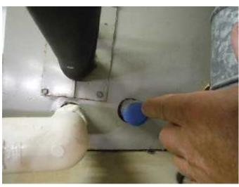
\* The lack of a secondary condensate drain piping or any moisture activated emergency shutoff switch will allow spilled condensate water to saturate and potentially damage building components under the garage installed air-conditioning evaporator coil. The lack of secondary condensate drain piping or a moisture activated emergency shutoff switch with an closet installed air conditioning evaporator coil does not meet minimum building standards and is a **NOT FUNCTIONING PROPERLY CONDITION**.
