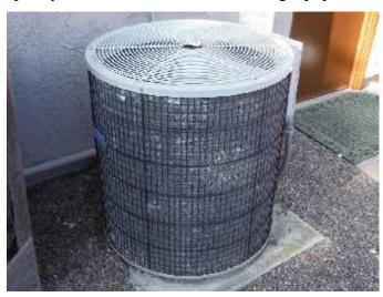
\* The split-system air-conditioner condensing unit and evaporator coil are older, have exceeded the expected service life, and even if serviced and repaired cannot be relied upon to continue to operate as intended. The older split-system air-conditioner equipment is an **END OF SERVICE LIFE - MATERIAL DEFECT CONDITION**.
