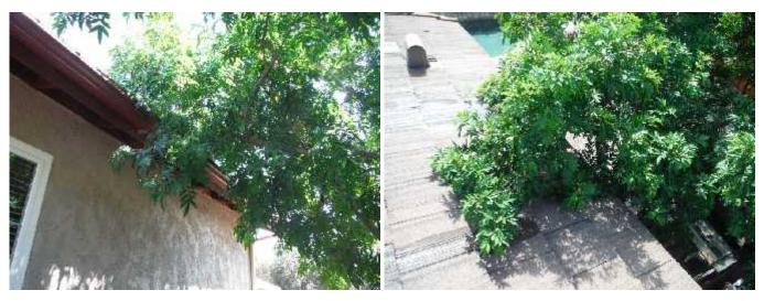
\* Vegetation extending over the building roof is continuously depositing leaf and branch debris onto this building's roof covering. Vegetation in contact with the building wall siding and trim will constantly convey moisture and contact abrasion to the building materials and is a **NOT FUNCTIONING PROPERLY CONDITION**.
