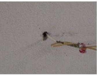
\* The annular gaps around the line-set and piping penetrations could allow a garage fire to seek oxygen through the open holes and spread into the dwelling attic structure. The openings through the garage fire-separation ceiling are a **SAFETY HAZARD CONDITION**.
