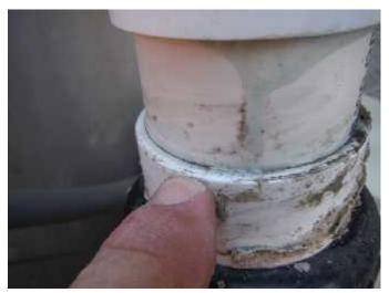
\* The leaking return piping will continue to leak wasting water until repaired. The leaking return piping is a **NOT FUNCTIONING PROPERLY CONDITION**.
