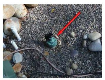
\* The lack of back-siphoning protection for the sprinkler control valve does not meet minimum safety standards and is a **SAFETY HAZARD CONDITION**.
