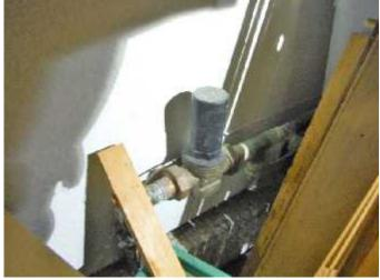
\* The water supply volume reduction with multiple faucets on, and the water pressure drop with only one faucet turned on indicates that the pressure regulator is not opening adequately when there is a demand for more volume as the regulator is designed to function. With the water volume drop with multiple fixtures on and the significant water pressure drop in the pressure regulator when one faucet is turned on is the pressure regulator device nearing an **END OF SERVICE LIFE CONDITION**.
