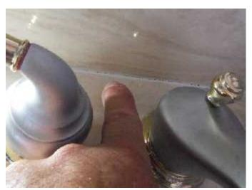
\* The open gap can allow moisture behind the countertop surface material into the cabinet / wall substrate which can swell from moisture saturation. The open separation between the bathroom countertop and backsplash material is a MAINTENANCE DEFICIENCY CONDITION.
