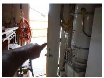
\* Doors accessing yards with pools and spa vessels through the interior must be self-closing and self-latching or contain alarms to prevent unattended access to a yard containing a pool or spa and potential drowning. The lack of an operating self-closing and self-latching mechanisms or alarms for the pool barrier-doors is a patent SAFETY HAZARD CONDITION.
