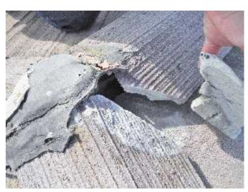
\* The deteriorated mortar on the end of the roof ridge is allowing moisture under the tile roof covering and onto wood the tile was meant to protect. The deteriorated ridge end mortar is an **END OF SERVICE LIFE CONDITION**.
