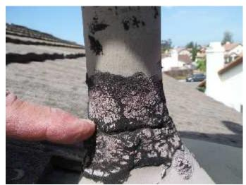
\* An open gap will allow moisture through the separation, below the roof penetration flashing, and into the roof deck assembly. The open separation gaps around the roof penetrations piping and the roof sheetmetal penetration flashings are an **END OF SERVICE LIFE CONDITION**.
