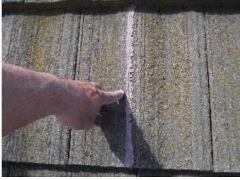
\* Minimum building standards find that roof tiles that are cracked or broken completely across the face of the tile in either direction shall be replaced. The gluing together of a broken (completely across the face of the tile) concrete roof tile is prohibited by building standards. Slipped roof tiles will continue to displace below the row of tiles and eventual expose the paper underlayment. The broken, glued together, and displaced tiles are a patent **NOT FUNCTIONING PROPERLY CONDITION**.
