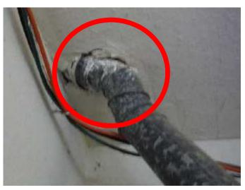
\* The water heater single-wall metal flue piping in contact with combustible materials (or within 6-inches of combustible materials) does not meet minimum safety building standards, is creating a potential fire hazard, and is a patent **SAFETY HAZARD CONDITION**.
