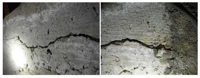
The south foundation stemwall east of the subarea crawlspace entry contains a horizontal crack that was not previously patched or repaired but is now cracked.
