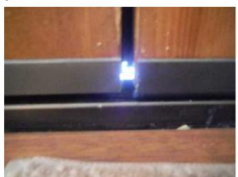
\* The missing weather-stripping will allow unheated air through the gap between the two doors and is a MAINTENANCE DEFICIENCY CONDITION.
