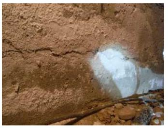
\* The reoccurring horizontal cracking indicates that there has been movement under the previous patching consistent with metal horizontal metal support (rebar) continuing to corrode and expand. The horizontal cracking that has not been patched, and cracking through the patching material on the foundation stemwalls will allow moisture in through the cracks and in contact with the stemwall interior metal support is a **NOT FUNCTIONING PROPERLY** — **MATERIAL DEFECT CONDITION**.
