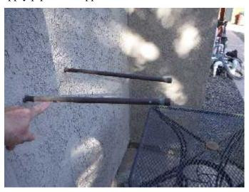
\* The protruding copper piping appears to have been in place for the addition of an exterior shower to rinse off pool water. The excessive protruding pipes are a potential impact hazard for some who does not se the piping when running around the corner of the building. The piping could rupture on impact or hurt someone from impact and is a **NOT FUNCTIONING PROPERLY CONDITION**.
