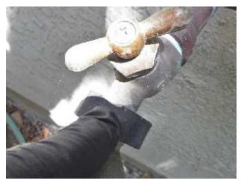
\* Modern safety standards require anti-siphon protection to be installed on all hose bib faucets to prevent cross-contamination of the potable water supply with water from attached hoses, and the lack of exterior hose bib faucet anti-siphon protection for the hose bib faucets does not meet minimum building standards, and is a potential **SAFETY HAZARD CONDITION**.
