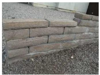
\* The masonry short wall was obviously damaged and was not repaired with mortar so the masonry blocks are just stacked upon each other and can easily fall. The substandard repair to the damaged masonry short wall is a **NOT FUNCTIONING PROPERLY CONDITION**.
