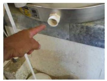
\* The lack of a drain piping extending down to the garage floor and away from the drywall covered water heater stand is a **MAINTENANCE DEFICIENCY CONDITION**.
