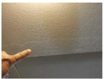
\* The improperly installed interior ceiling patch around the attic access hatch is a **NOT FUNCTIONING PROPERLY CONDITION**.
