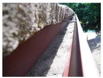
\* The height of the upper roof rain gutters precludes someone cleaning them without adequate training and the proper equipment. The debris filled roof rain gutters are a **NOT FUNCTIONING PROPERLY CONDITION**.
