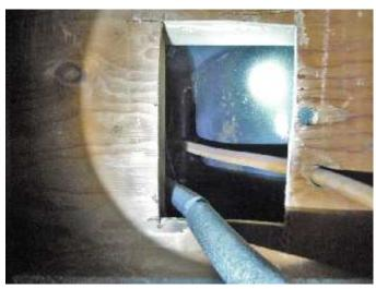
\* The lack of a protective covering over the opening to restrict access to the interior wall adjacent to the bathtub can allow rodents and other vermin into the interior of the bathroom walls and does not meet minimum building standards and is a **NOT FUNCTIONING PROPERLY CONDITION**.
