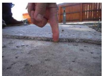
\* The broken walkway with height differential that is a possible trip hazard is a **SAFETY HAZARD CONDITION**.
