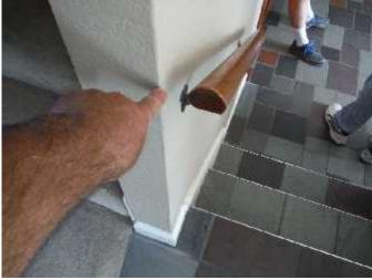
\* With the handrail end projecting outward a sleeve can get caught in the exposed handrail end - causing a trip hazard. The exposed handrail end does not meet minimum safety standards and are a patent **SAFETY HAZARD CONDITION**.
