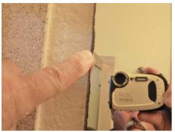
\* The damaged reflective backing will continue to corrode until replacement is warranted and is an **END OF SERVICE LIFE CONDITION**.
