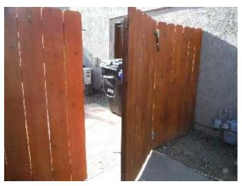
\* City of San Diego minimum health and safety requirements for protective barriers to prevent drowning requires that all gates accessing yards with pools be self-latching to prevent unattended access to a yard containing a pool. The lack of self-latching barrier gates for the pool / spa area does not meet minimum safety standards to prevent child drowning. The improperly not self-latching gate is a patent **SAFETY HAZARD CONDITION**.
