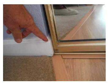
\* The constant hitting of the interior sliding mirrored closet doors to their running baseboard molding can eventually cause the mirrored glass to shatter. The missing door bumpers are a **SAFETY HAZARD CONDITION**.
