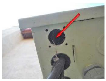
\* The open knockout in the bottom of the accessible electrical panel box can allow access into the inner electrical panel components which are electrically energized and could be inadvertently accessed by someone interfacing with the electrical panel. The open knockout in the electrical panel exterior box does not meet minimum safety requirements and is a patent SAFETY HAZARD CONDITION.
