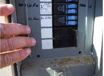
\* The lack of labeling for each circuit's use will inhibit repair and emergency access when shutting off a specific electrical circuit. The lack of labeling for each electrical circuit's use does not meet minimum modern building and safety standards, and is a patent **SAFETY HAZARD CONDITION**.
