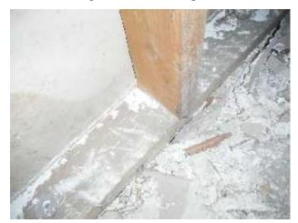
\* Drawing unfiltered air into the forced-air conditioned air stream adds pollutants directly into the interior of the dwelling and the equipment interior heat-exchanger. The open holes and gaps through the return-air wall framing does not meet minimum building and safety standards and is a **NOT FUNCTIONING PROPERLY CONDITION**.
