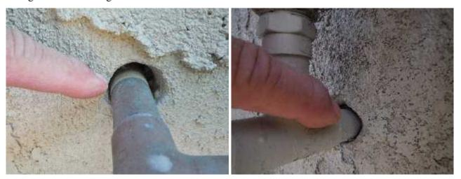
\* The open annular gaps around penetrations and small cracks through the exterior wall covering can allow moisture through the exterior wall covering and are a **MAINTENANCE DEFICIENCY CONDITION**.
