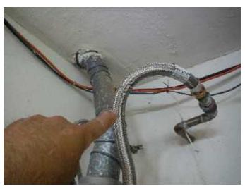
\* The lack of insulation on the hot and cold water lines allows heat to dissipate directly from the warmer upper portion of the tank lowering the efficiency of the heated water. The lack of insulation on the water heater water lines, as required by the manufacturer and minimum building standards, is a patent **NOT FUNCTIONING PROPERLY CONDITION.**
