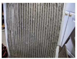
\* The dirty air-filter will inhibit air flow to the furnace heat-exchanger causing the heat-exchanger metal to overheat air filter is an **END OF SERVICE LIFE CONDITION**.
