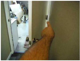
\* The damaged fire-rated door would provide oxygen to a garage interior fire thus spreading the fire into the interior of the dwelling. The modified fire-rated door is a patent **SAFETY HAZARD CONDITION**. The lack of 2-spring hinges required for self-closing and self-latching the fire-rated door between the attached garage and the dwelling interior does not meet minimum safety standards and is a patent **SAFETY HAZARD CONDITION**.
