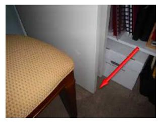
\* The lack of functioning floor-guide for bedroom bypass closet doors allows the doors to protrude or bind from swinging outward or inward during their operation and is a **MAINTENANCE DEFICIENCY CONDITION**.
