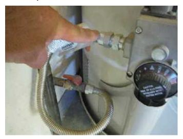
\* The absence of a sediment trap on the gas piping for the water heater does not meet Manufacturer's installation requirements thus potentially voiding warranty coverage, the building standards applicable when the manufacturing of the appliance occurred, and is a patent **SAFETY HAZARD CONDITION**.
