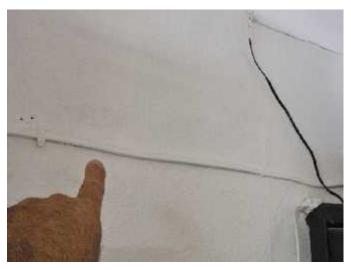
\* Accessible exposed horizontal wiring in garages is prohibited by building standards to protection children from being in contact with damaged electrical wiring while pulling or climbing on the exposed wiring. The lack of adequate protection for the Nonmetallic Sheathed Cable (Romex) does not meet minimum building and safety standards and is a SAFETY HAZARD CONDITION.
