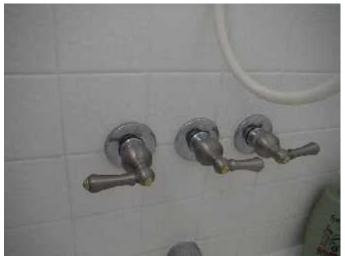
\* The 3-handled shower faucet valves do not offer single-valve thermal protection like modern single-stem faucets offer and is an **END OF SERVICE LIFE CONDITION**.
