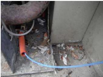
\* The reason for the pool / spa water heater to not function as intended is not self-evident but there is rodent nesting material in the burn chamber of the water heater. The operation of the natural-gas pool / spa water heater is an UNKNOWN CONDITION AND DEFERRED.
