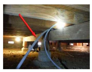
\* The abandon water supply piping not cut back to the point where the plastic piping penetrates the floor construction and then removed is an unfinished installation of the re-piping installation and is a **MAINTENANCE DEFICIENCY CONDITION**.
