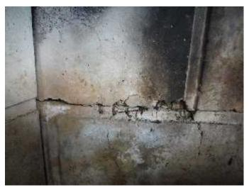
\* The cracked refractory plates are no longer functioning as initially intended. The cracked refractory plates are a **NOT FUNCTIONING PROPERLY CONDITION**.
