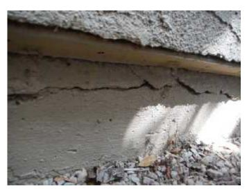
The north wing of the kitchenette popout walls has a horizontal crack. This area of the kitchenette popout section of the east perimeter foundation and building wall was not previously patched.
