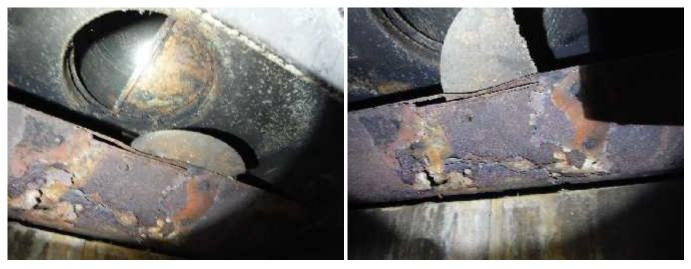
\* The extensive damage to the metal firebox throat area is a patent **SAFETY HAZARD – MATERIAL DEFECT CONDITION**.
