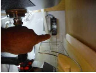
\* Electrical conductors are required to be enclosed in sheathing or conduit for the protection of the wire insulation. The exposed conductors feeding the lighting transformer should have been run in a cord or conduit protection until into the transformer body, does not meet minimum safety standards and is a **SAFETY HAZARD CONDITION**.
