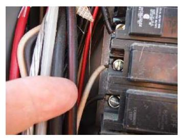
\* The use of a white wire is prohibited by minimum building standards in order to reduce the risk of someone contacting the white wire assuming it is as still neutral conductor. The white wire being used as a hot conductor and no properly codded as no longer a neutral and is a **NOT FUNCTIONING PROPERLY CONDITION**.
