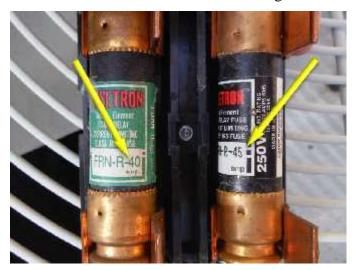
\* The different amperage fuses for the exterior condensing unit does not meet the minimum manufacturer requirements, could void the manufacturer warrant coverage for the condensing unit equipment, could damage the condensing unit electrical components by not supplying the needed amperage the condensing unit needs to operate properly, and is a patent **NOT FUNCTIONING PROPERLY CONDITION**.
