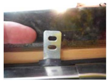
\* The built-in dishwasher needing to be secured to the cabinet structure is a **NOT FUNCTIONING PROPERLY CONDITION**.
