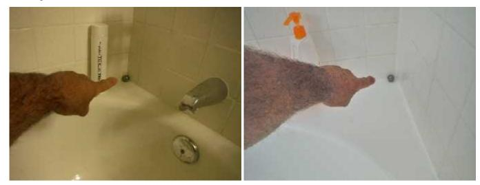
\* With water sitting on the bathtub rim there is potential for moisture to migrate under the shower enclosure walls and come in contact with the wall materials behind the shower enclosure walls. The improperly sloped bathtub rim does not meet minimum installation requirements for draining all shower spray to the bathtub vessel drain and is a MAINTENANCE DEFICIENCY CONDITION.
