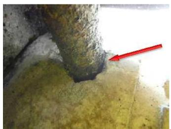
\* The open gap around the gas piping could allow heat to draft through the annular opening and into the components behind the firebox side refractory plate wall. The annular separation around the gas piping does not meet Manufacturer requirements and is a **SAFETY HAZARD CONDITION**.
