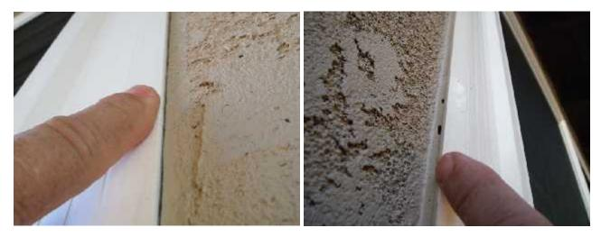
\* The 'Easy-Framed' windows on the exposed exterior walls will need periodic sealant applied to the top and two sides (not the bottom) to control moisture from entering behind the exterior window phalange. is a **MAINTENANCE DEFICIENCY CONDITION**.
