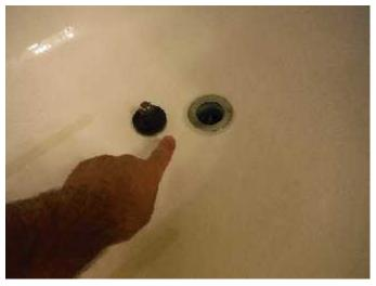
\* The damaged bathtub drain screw-in drain stopper assembly can no longer be relied upon to function as intended and is an **END OF SERVICE LIFE CONDITION**.
