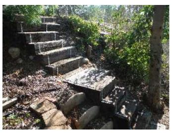
\* Exterior stairway without handrail protection does not meet minimum safety and building standards and presents a potential fall hazard for a user of the stairs out of balance while descending the stairway. The lack of handrail for a stairway with 4 or more risers is a patent **SAFETY HAZARD CONDITION**.
