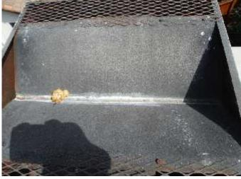
\* Water is held around the flue penetration and eventually will corrode the sheet-metal cap allowing moisture into the chimney chase structure to damage the fireplace components. The improperly sloped chimney termination cap is a **NOT FUNCTIONING PROPERLY CONDITION**.
