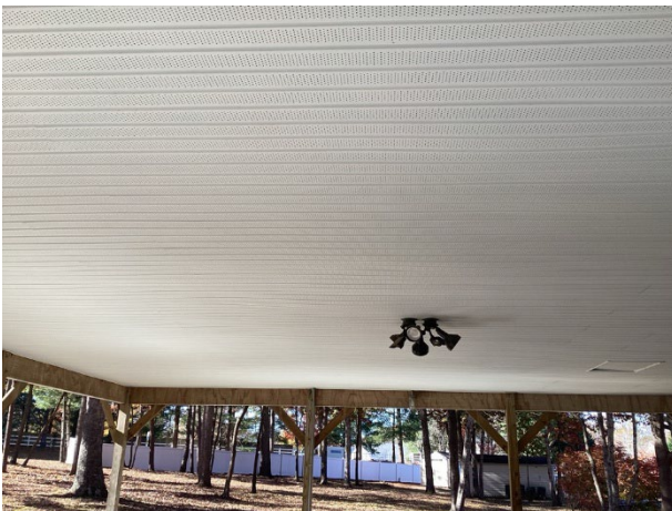
Soffit and light fixtures at pavilion
