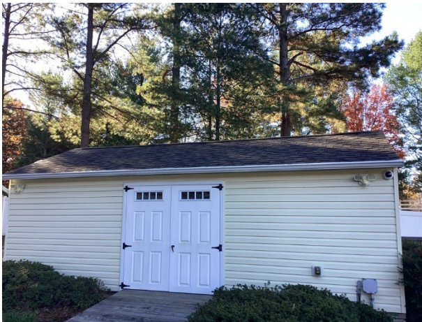
Shed roof overview
