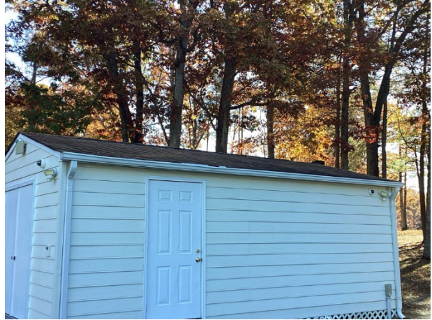
Shed roof overview
