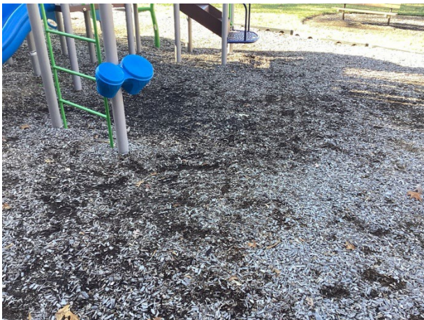
Safety surface depletion
