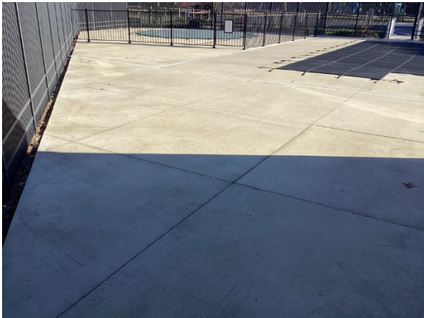
Concrete pool deck overview
