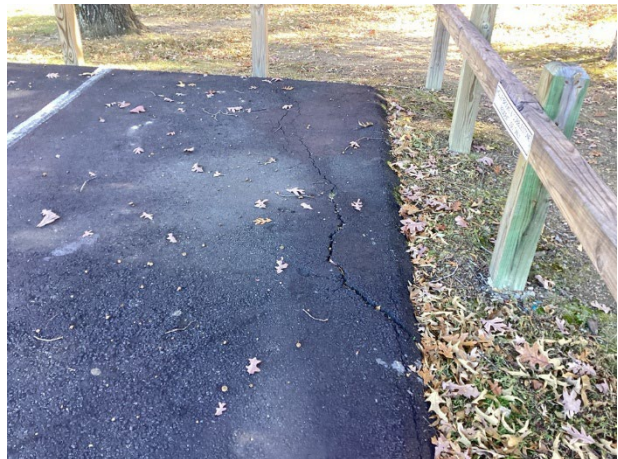
Pavement cracks
