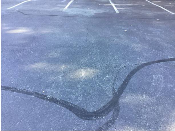
Pavement cracks
