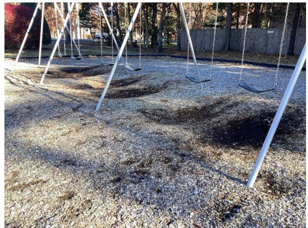
Safety surface depletion
