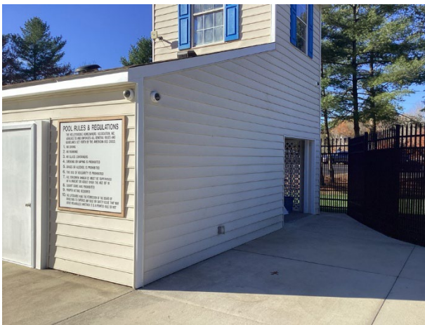
Vinyl siding overview
