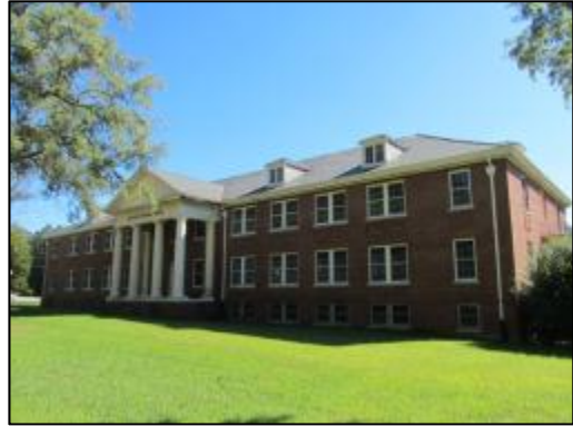
NCDOT Survey #41, Galen Stone Hall, Palmer Memorial Institute Historic District (GF-0180), looking northeast.
