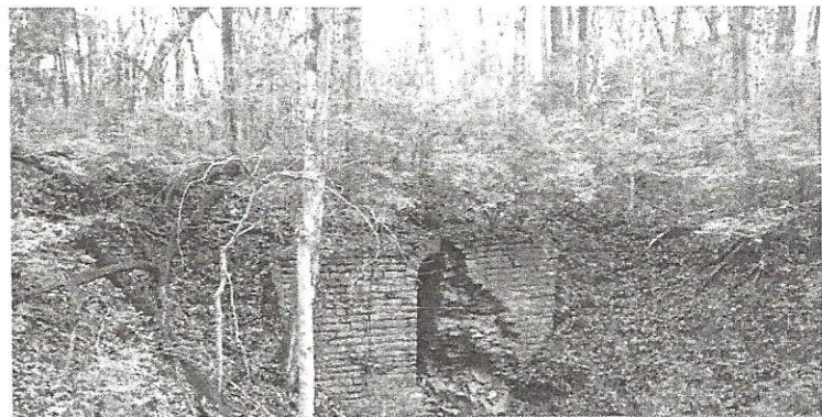
Existing culvert remains from former "Swing Line" interurban rail
