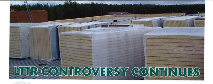
CAN/ULC-S770, Standard Test Method for Determination of Long-Term Thermal Resistance (LTTR) of Closed-Cell Thermal Insulating Foams, was developed to predict the R-values of rigid closed cell plastic foam insulations. It is widely accepted that the thermal resistivity of closed cell insulations that rely on captive blowing agents decreases over time before it stabilizes. The test method in S770 is used to predict the magnitude of this change in the R-value.
