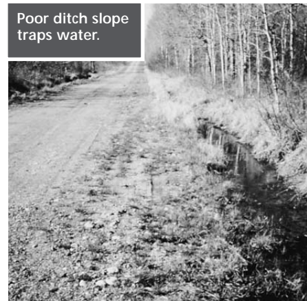
Shallow and narrow ditch. Likely to cause road flooding and future damage.
