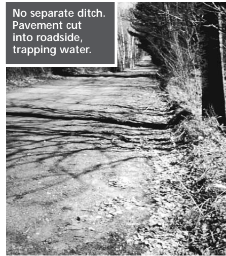
Poor ditch slope traps water.
