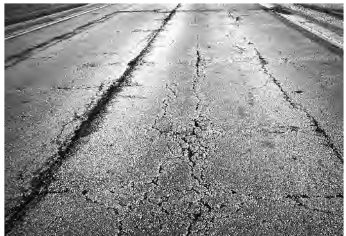
Multiple open, longitudinal cracks that are raveling. ▼
