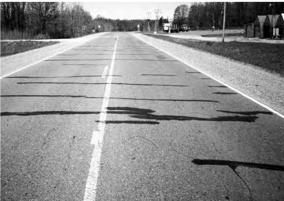
◀ Sealed cracks, a few feet apart.
