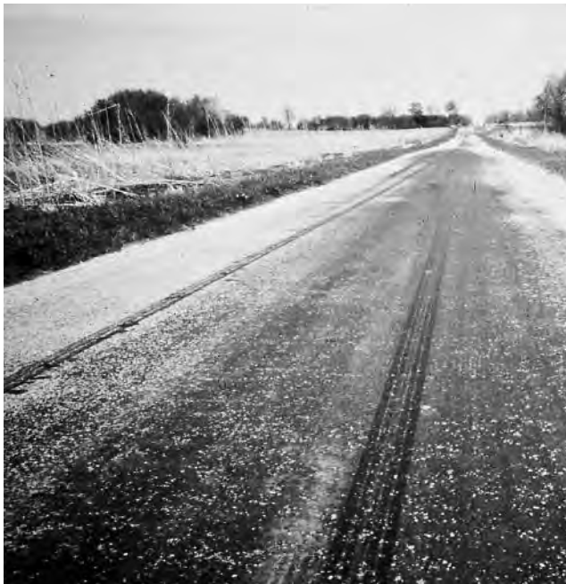
▼ Severe flushing.
