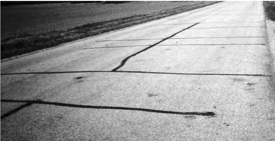
▼ Open crack, 1/2" wide; adjoining pavement sound.
