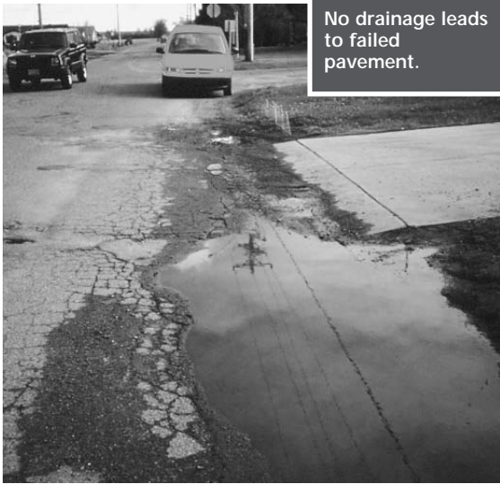
High water has damaged pavement.
