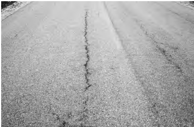
Multiple open, longitudinal cracks that are raveling. ▼
