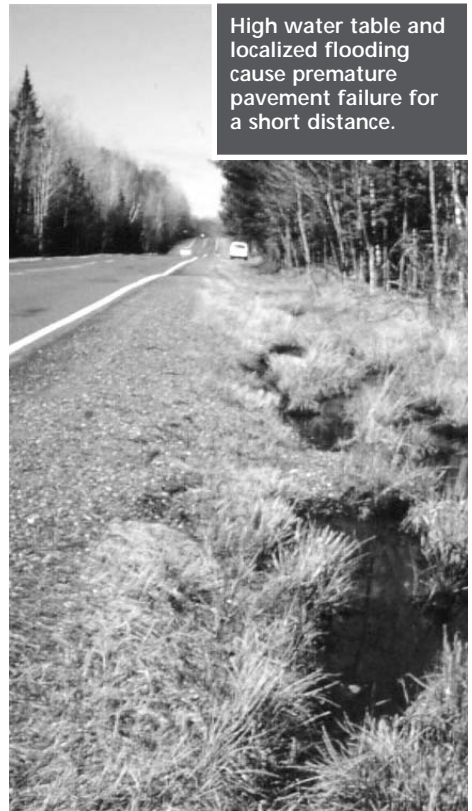
Secondary ditch traps water. Actual ditch adequate. Minor grading will restore crown and drainage.
