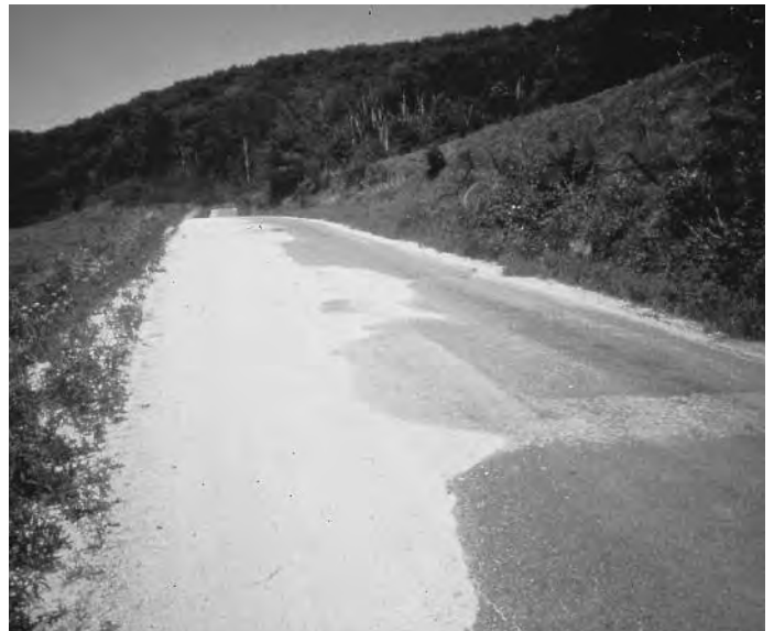
▲ Wedges and patches extensive but in good condition.
