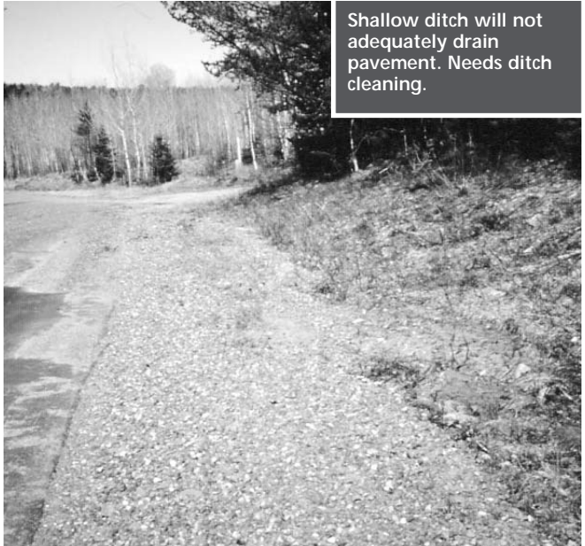
Secondary ditch traps water. Actual ditch adequate. Minor grading will restore crown and drainage.
