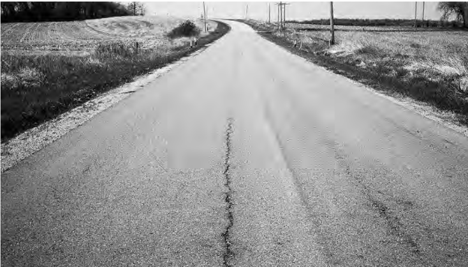
▼ Slight rutting; patch in good condition.
