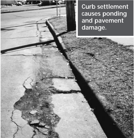
Lack of positive gradient causes flooding.
