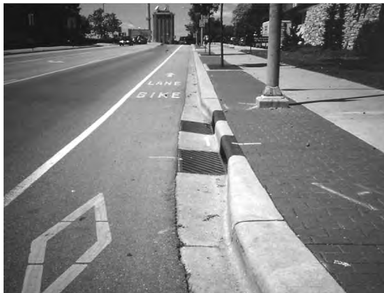
Urban drainage. RATING: Excellent
