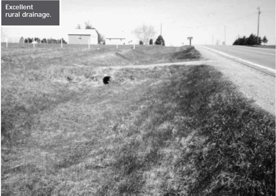
Excellent culvert and end protection.
