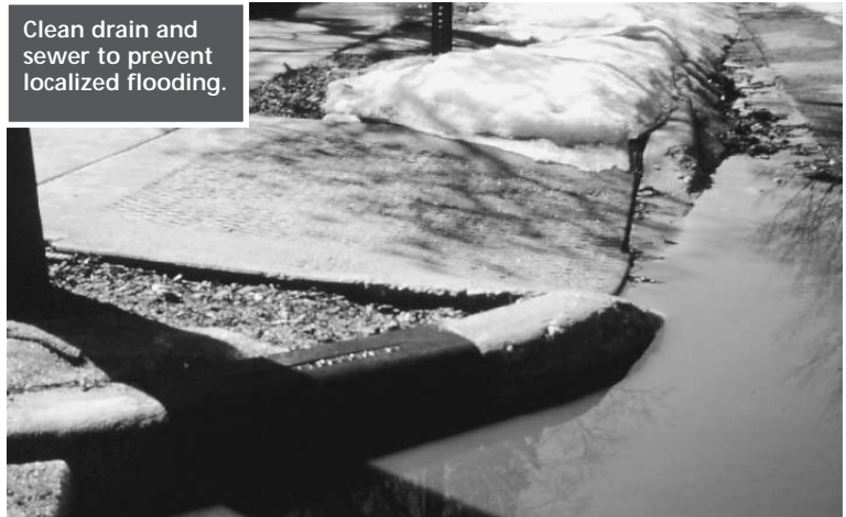
Reshape terrace behind curb to restore drainage and prevent damage to curb and street.
