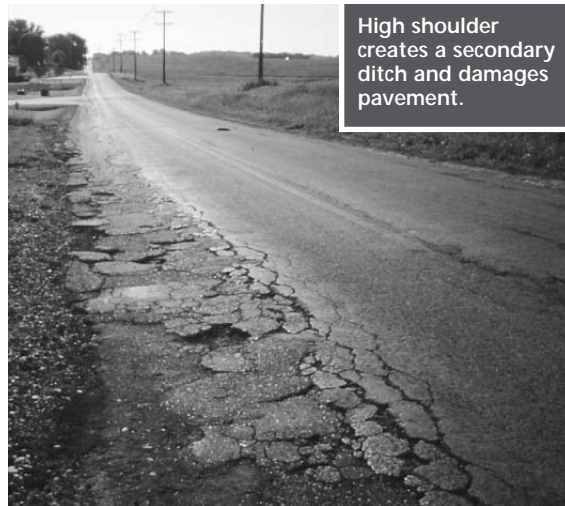
No separate ditch. Pavement cut into roadside, trapping water.
