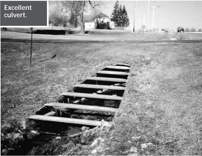
Excellent culvert and end protection.
