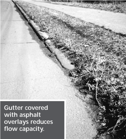
Silt from adjacent property causes flooding.
