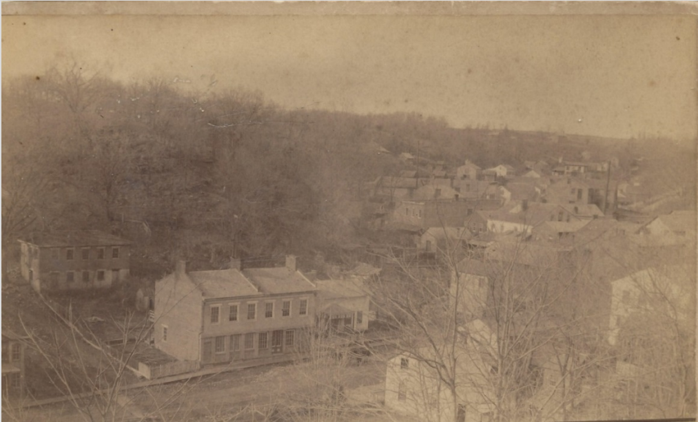
Main St. Running Horizontally Into The Town Of Galena, Illinois
