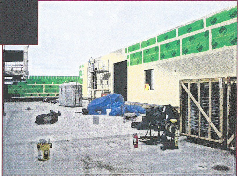
Photo 2 – Application of liquid-applied WRB.
