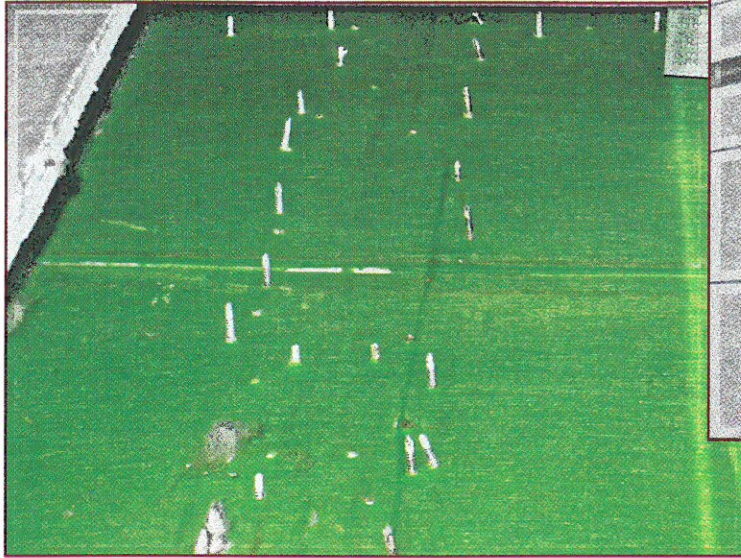
Photo 8 – Fasteners missing studs.
