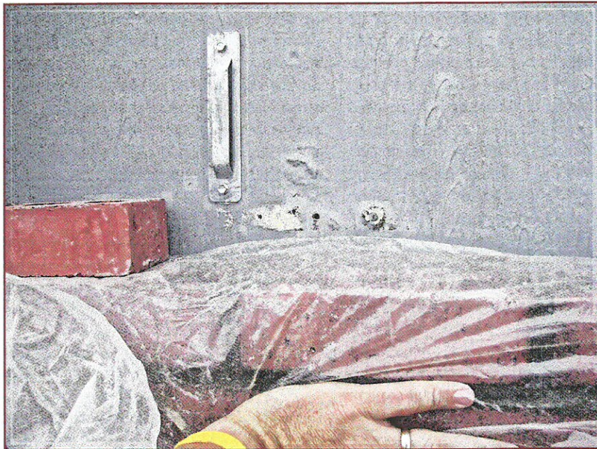
Photo 12 – Multiple holes in WRB.
