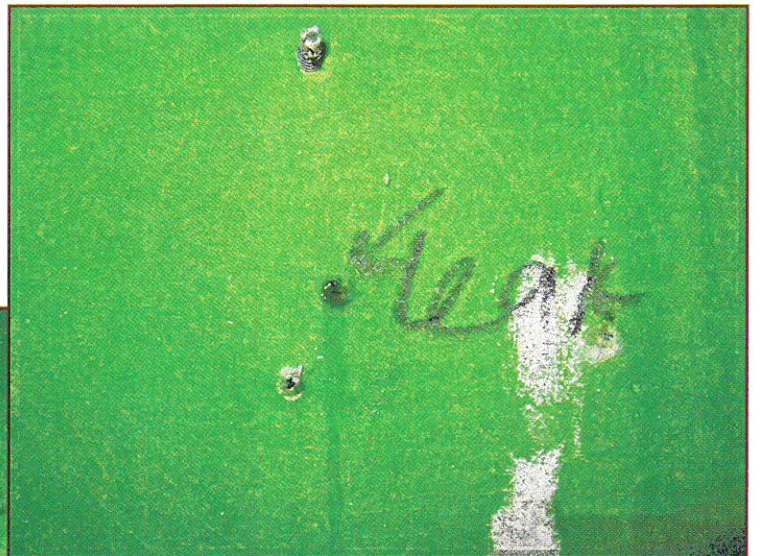
Photo 11 – Water leak at missing fastener hole in gypsum sheathing.
