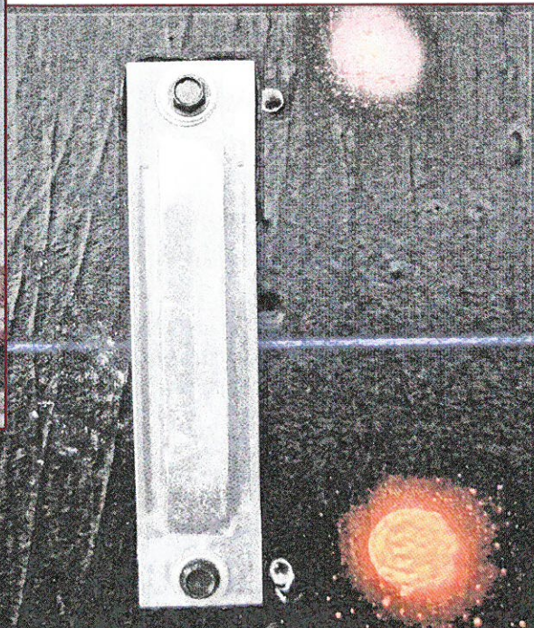
Photo 13 – Holes in WRB adjacent to brick tie.
